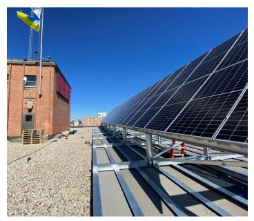
MMF building could support 168 solar panels, generating up to 73 kW of solar electricity for the building.
