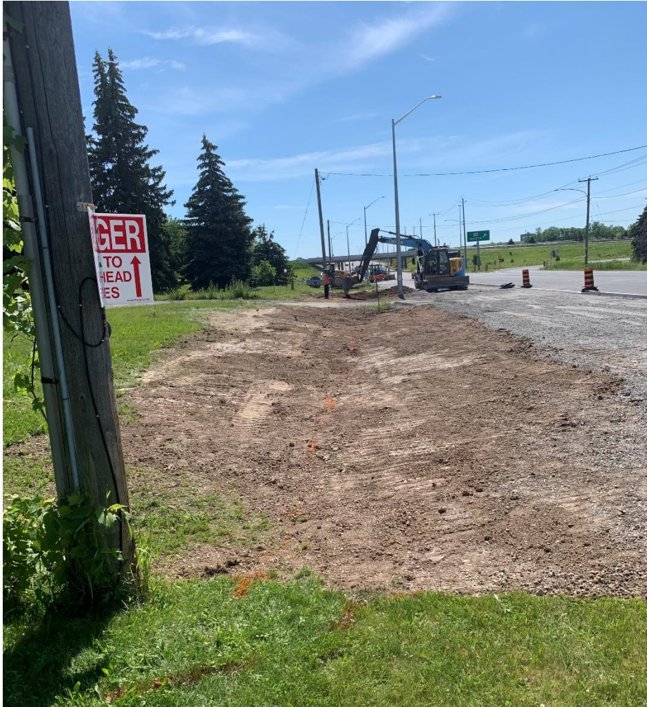
Excavating for Drainage Improvements
