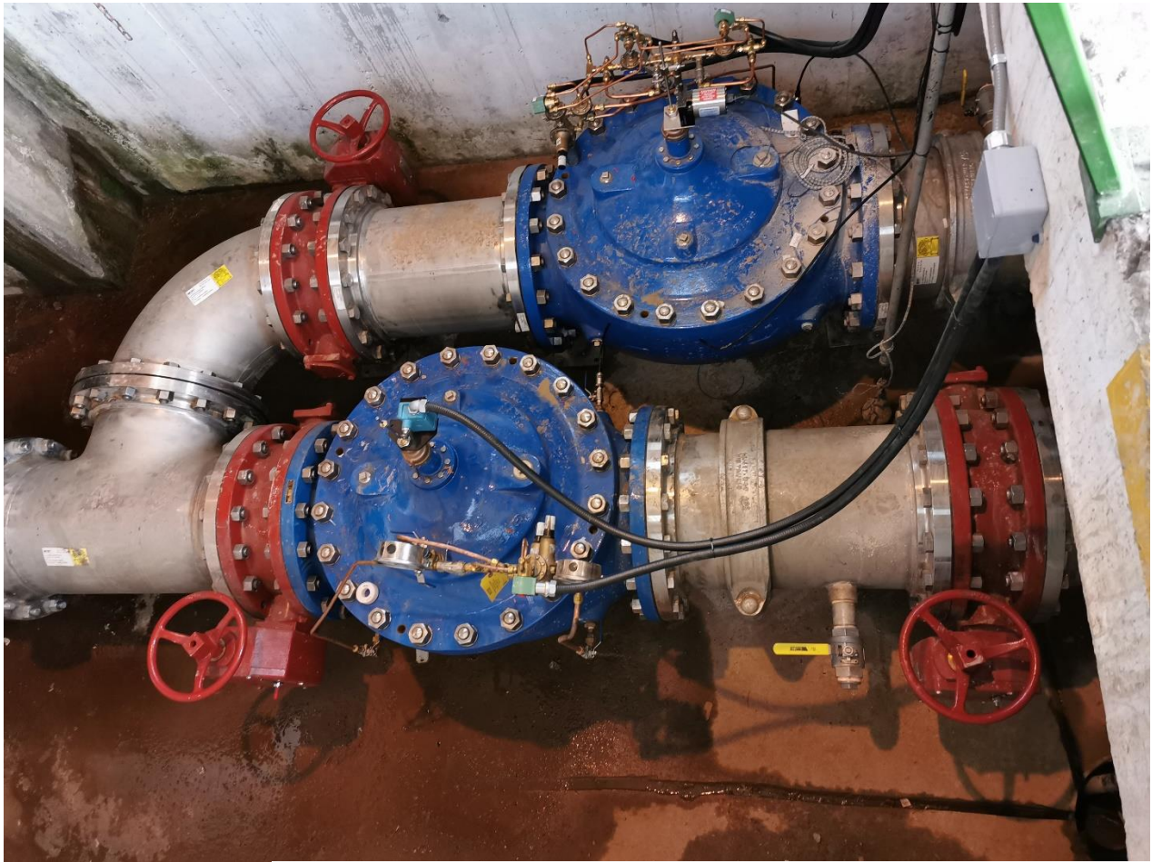
Complete Installation of Dual Stage Pressure Reducing Valves
