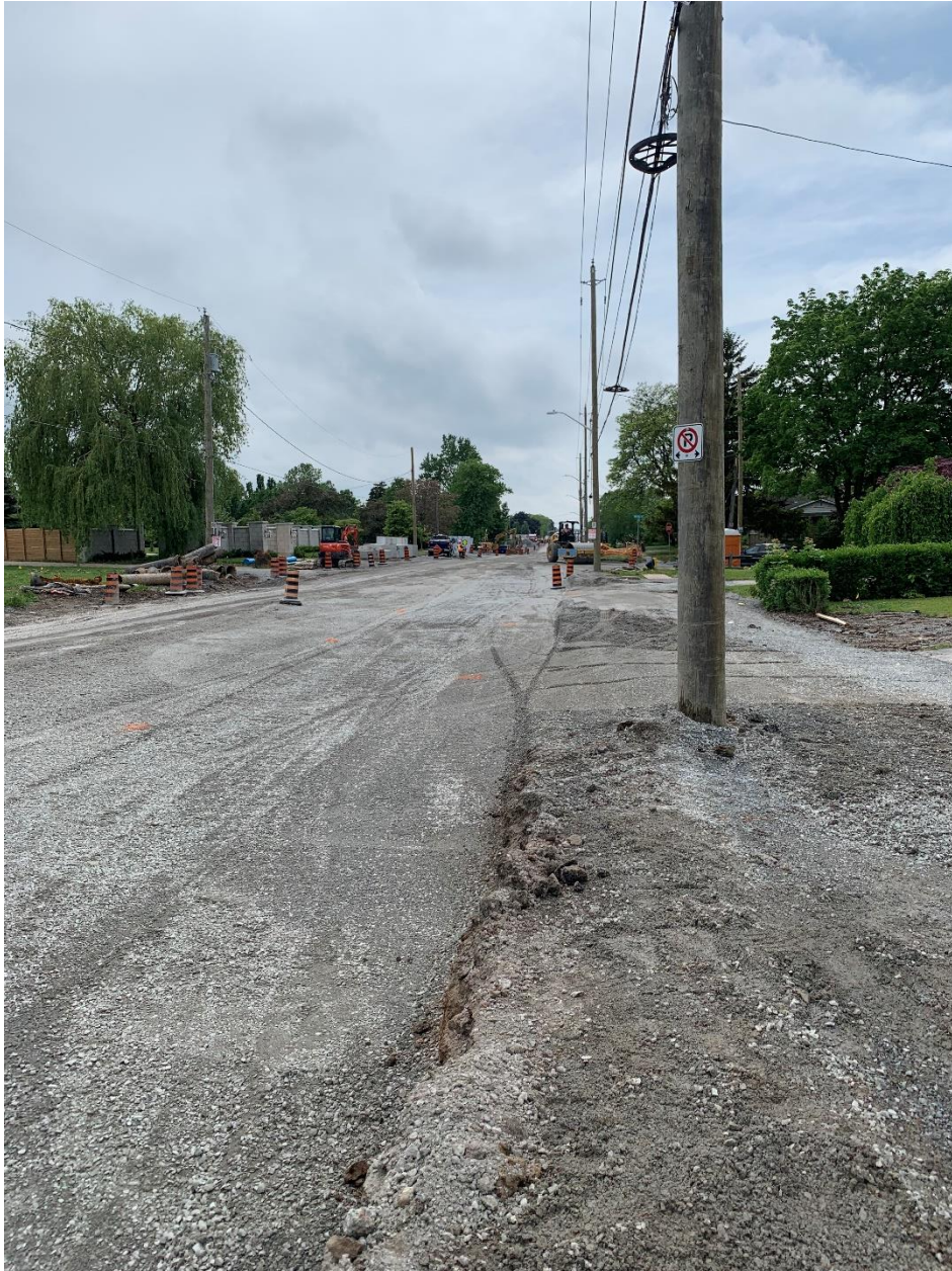
Initial Grading of Road Subgrade
