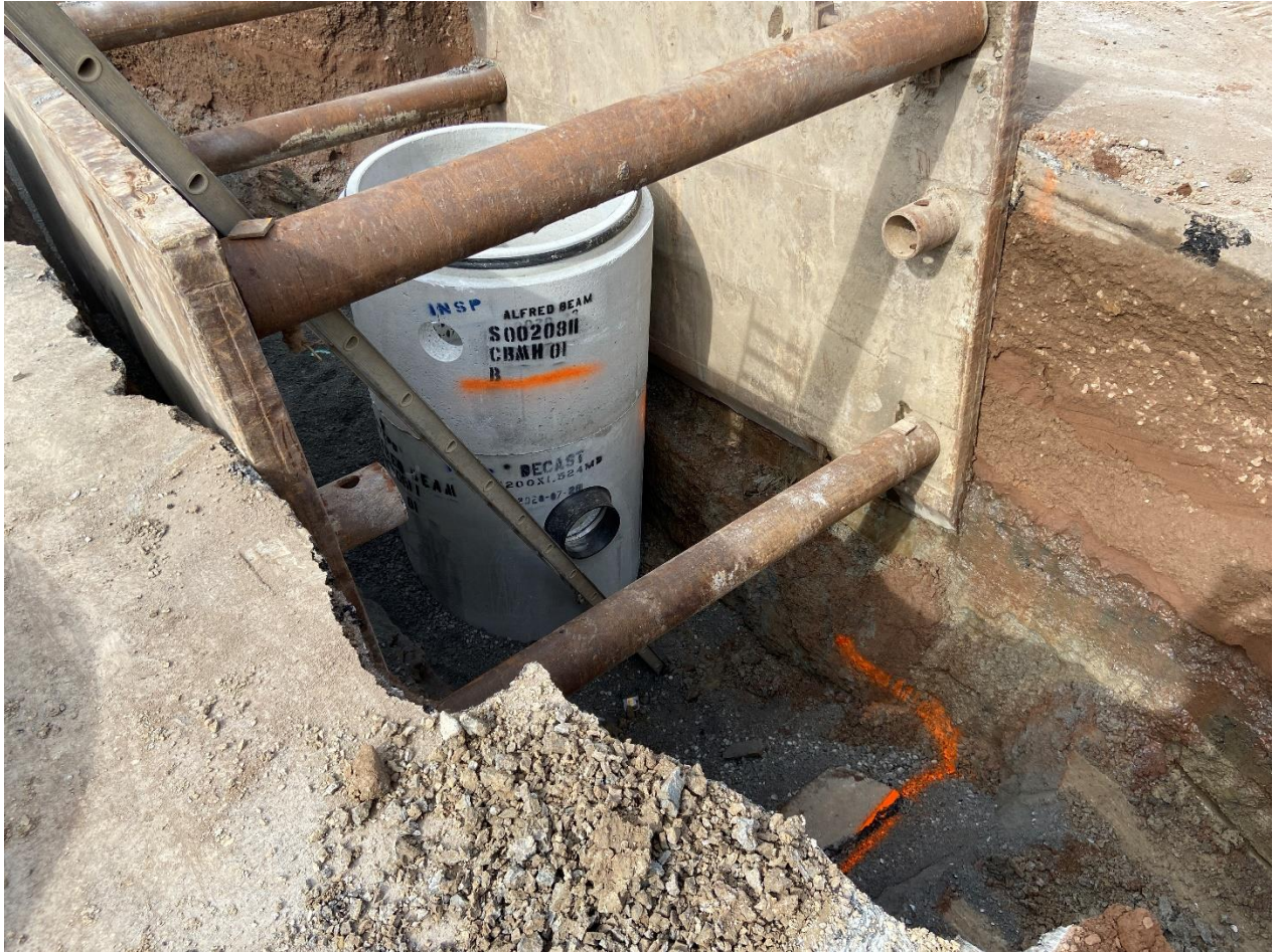
Maintenance Hole Installation
