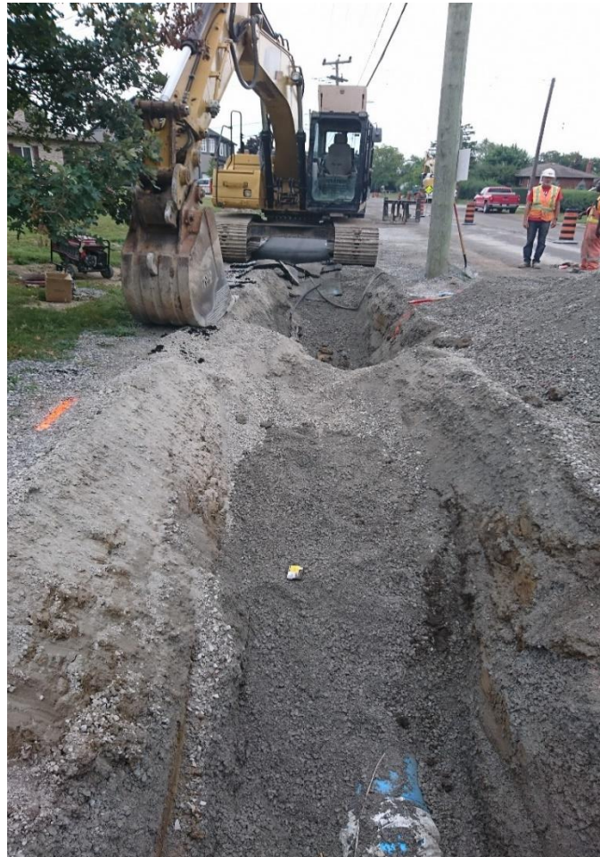
Figure 3: Watermain Installation
