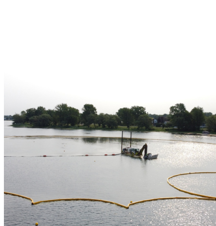
Silt curtain sequesters sediment during dredging operation
