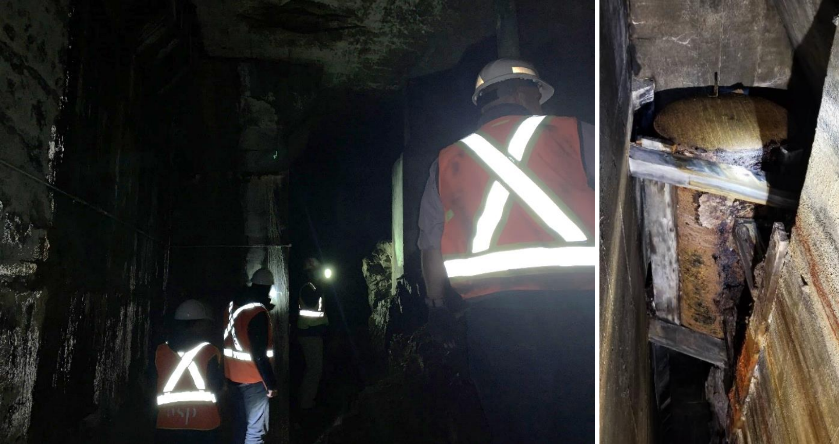
Figure 3: Sub-surface cavity beneath the Iqaluit WTP known as the Void (left) and a 60-year old abandoned underground fuel storage tank (right)
