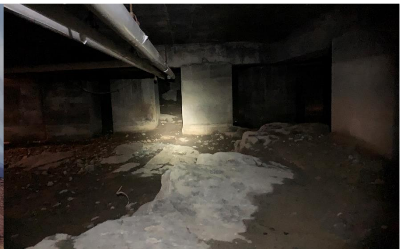
Figure 6: Removal of the historic underground fuel storage tank (left) and the Void after cleaning (right)..
