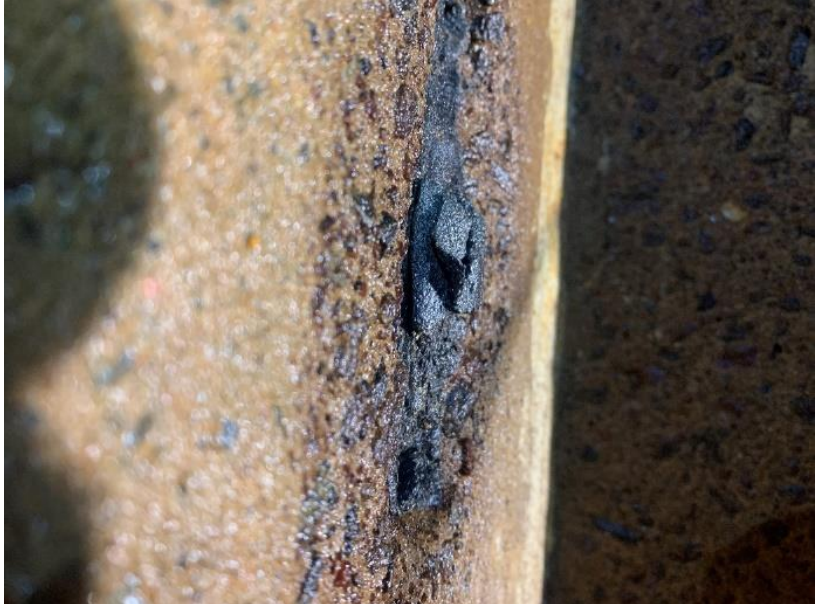
Figure 7: Iqaluit Water Treatment Plant below-ground tank inspections and black tar-like substance
