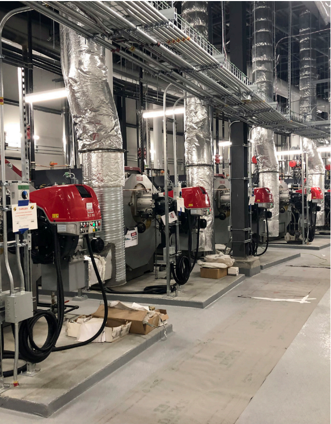
Image 16: High efficiency dual fuel condensing boilers © Ross Griffiths, Arup
