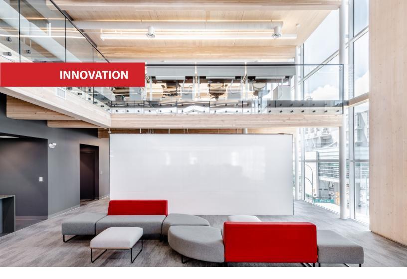
Fast + Epp's home office building uses hybrid mass timber and steel as the structure's fundamental building block to demonstrate material efficiency, cost-effectiveness, and sustainable construction.
