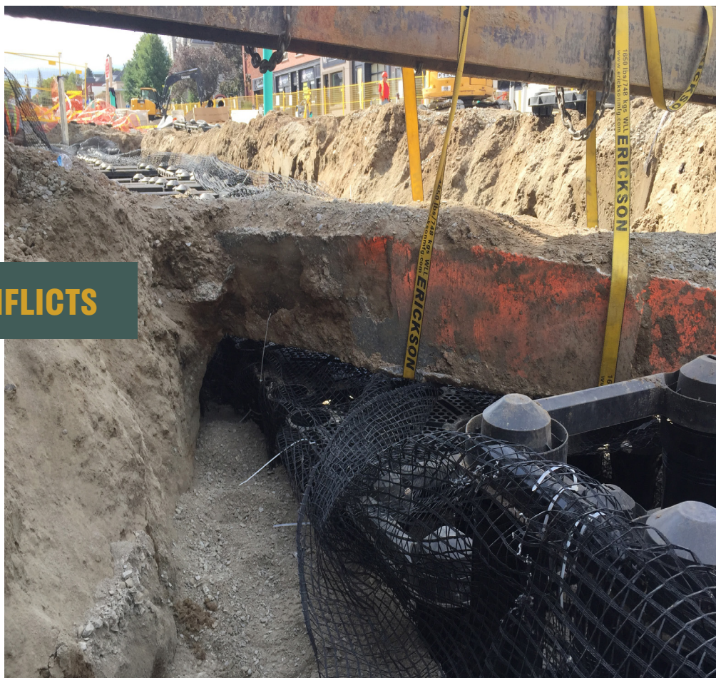
FIGURE 8: SUPPORTING UTILITIES DURING INSTALLATION OF SILVA CELLS
