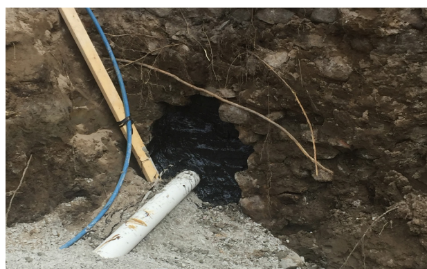
FIGURE 12: STORM SEWER THROUGH FOUNDATION WALL
