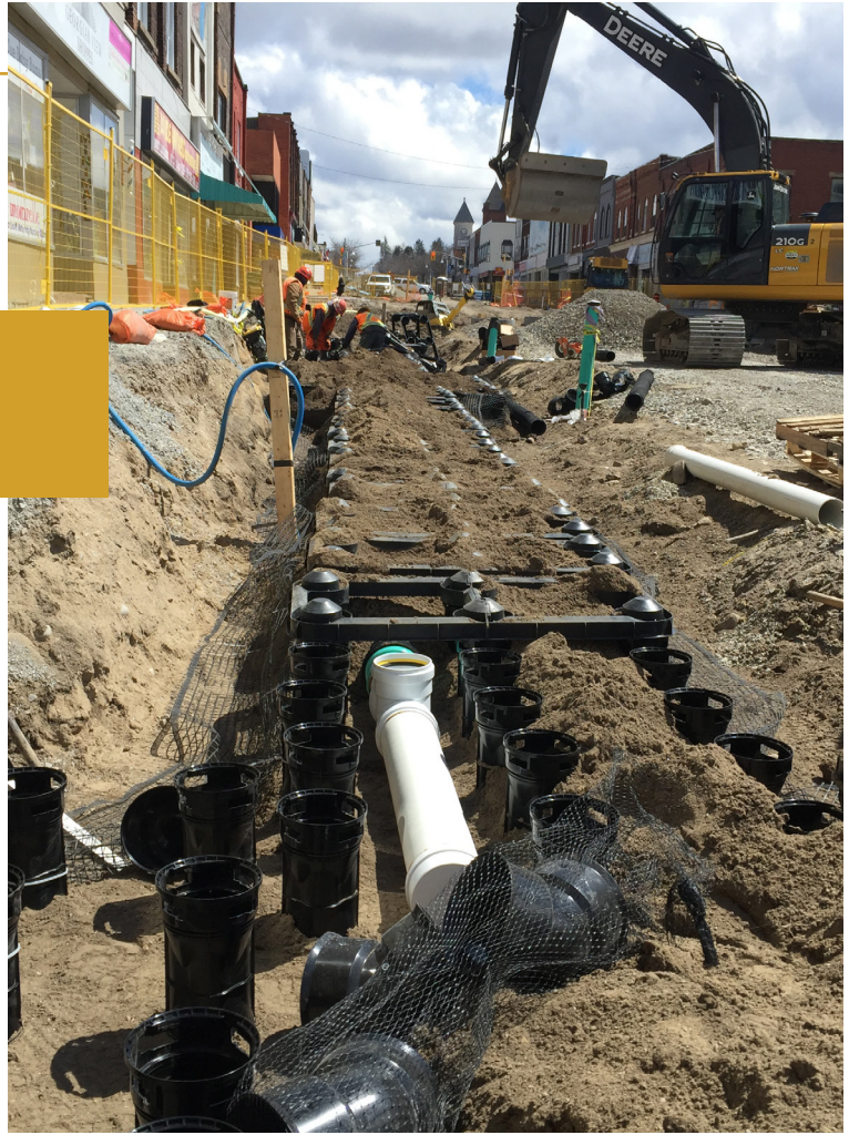
FIGURE 5: CONSTRUCTION OF SILVA CELL SYSTEM
