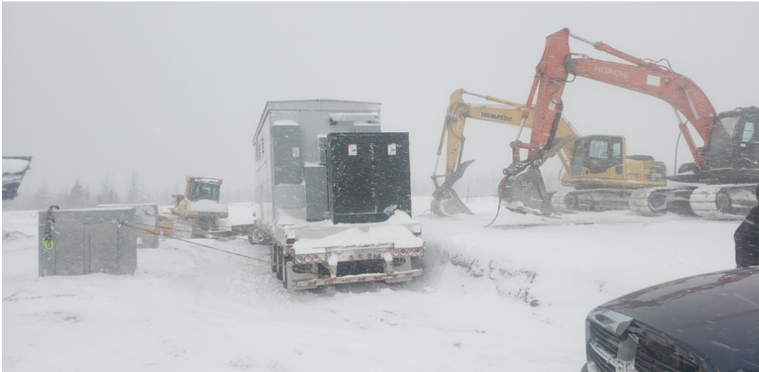
Image: E-house installation during a blizzard
