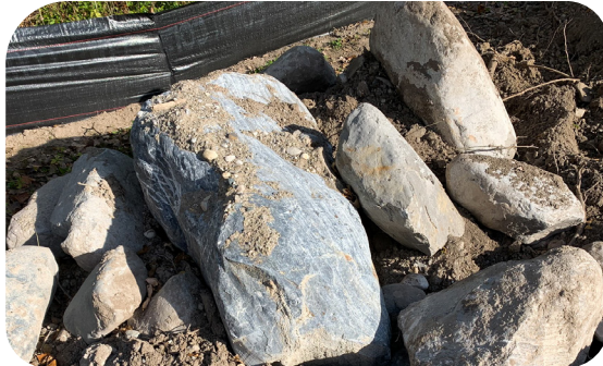
Boulders encountered while driving sheet piles for the stay-in-place cofferdams
