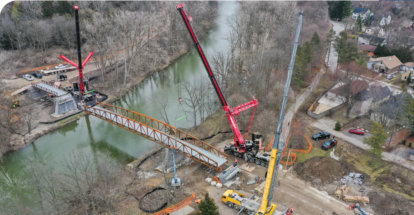
Below: Ross Park Bridge centre span being erected using two cranes in tandem
