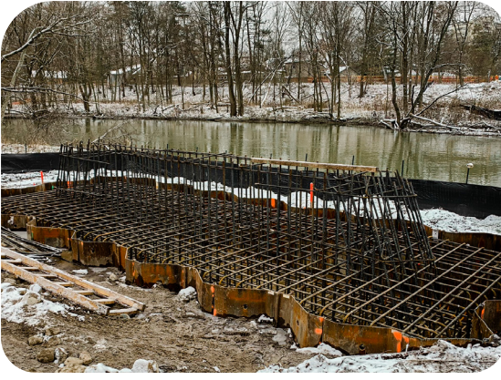
Pier foundation with stay-in-place sheet pile cofferdam adjacent to the North Thames River
