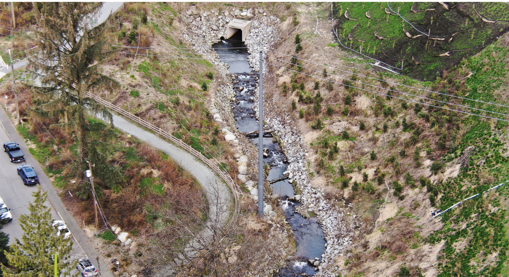
New Keith Creek channel with fisheries habitat enhancements.
