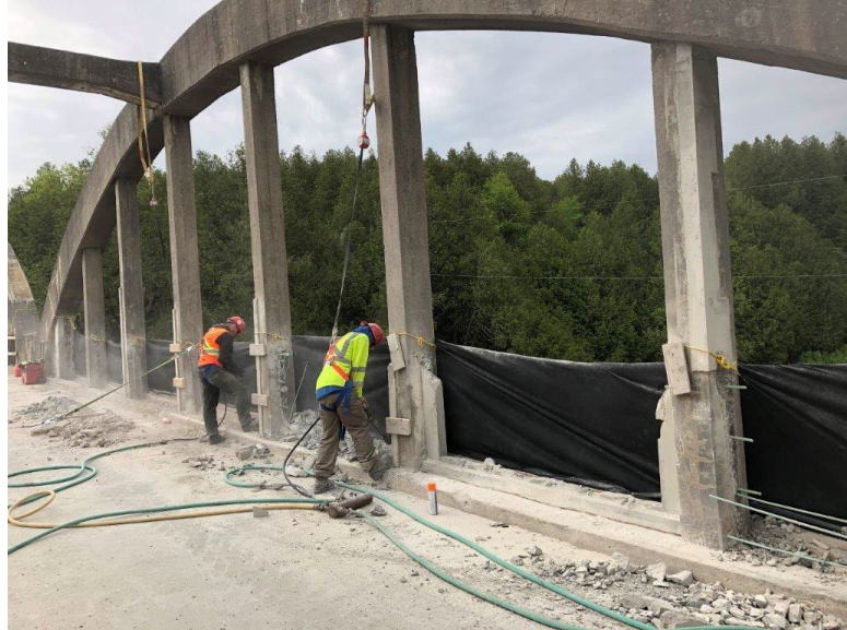
Image 5: Removal of Existing Deck
