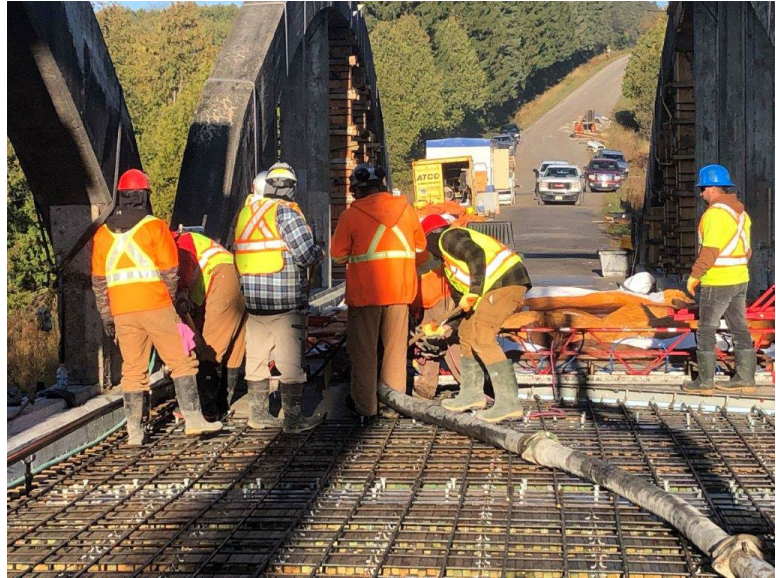
Image 8: Installation of Concrete Composite Deck
