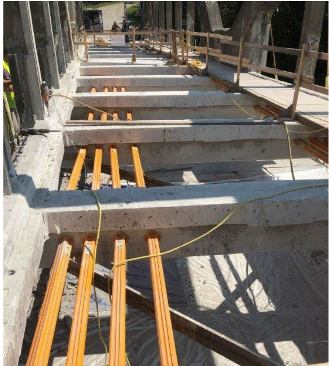
Image 6: Temporary Deck Struts Installed for Buckling Prevention
