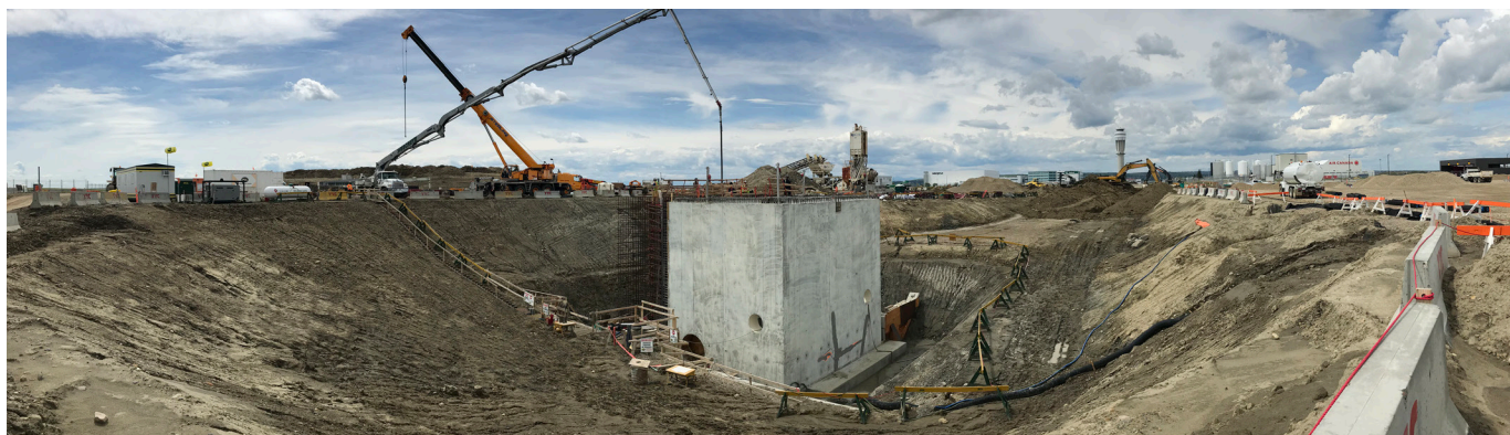
Open Excavation of the Diversion Structure
