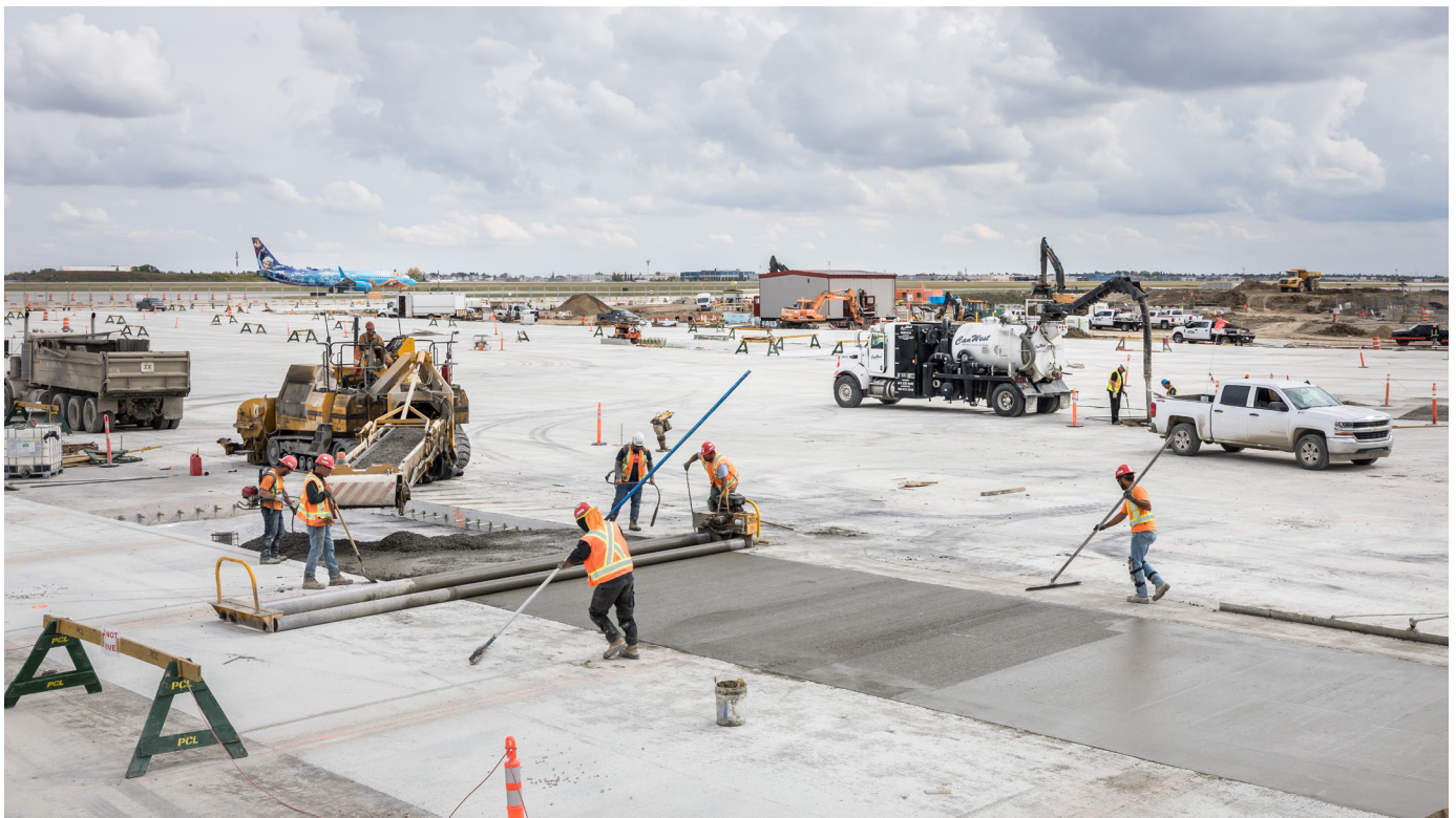
Concrete Apron Construction
