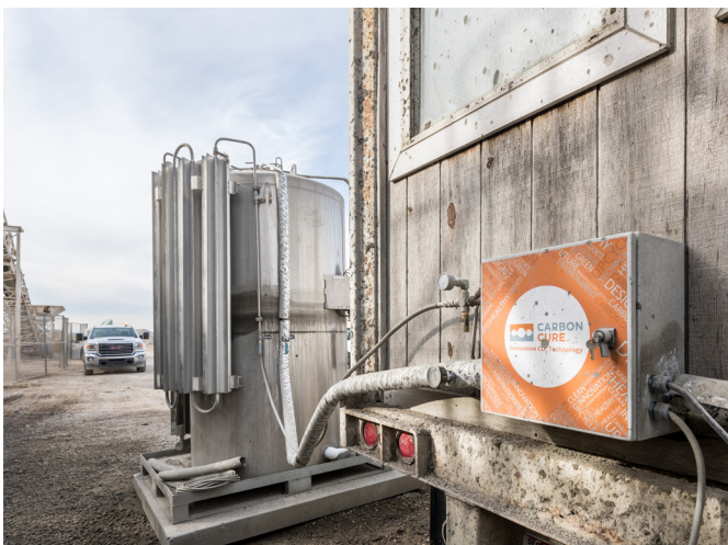
Industrial Waste Carbon Dioxide Tank
