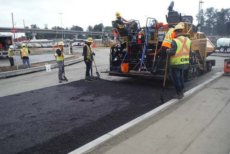
Asphalt Paving
