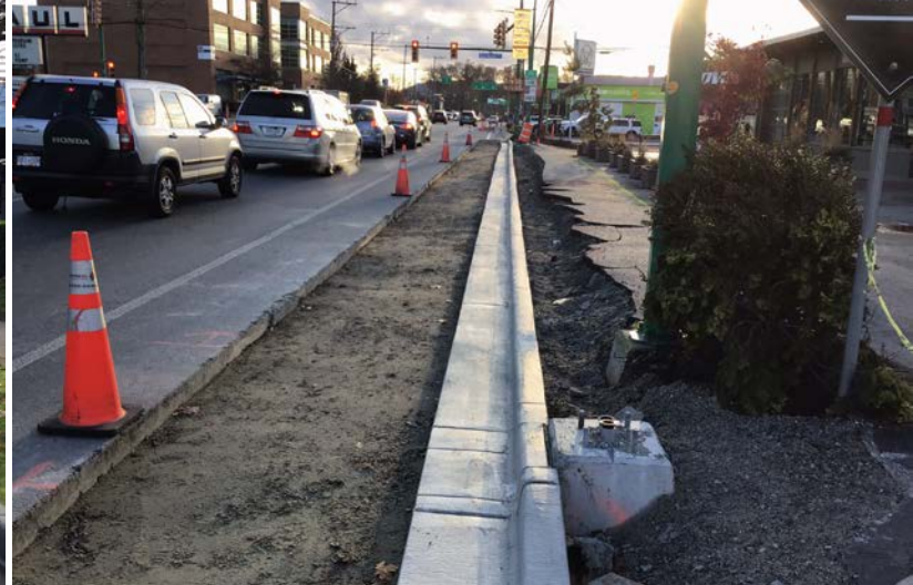
New curb and gutter installation
