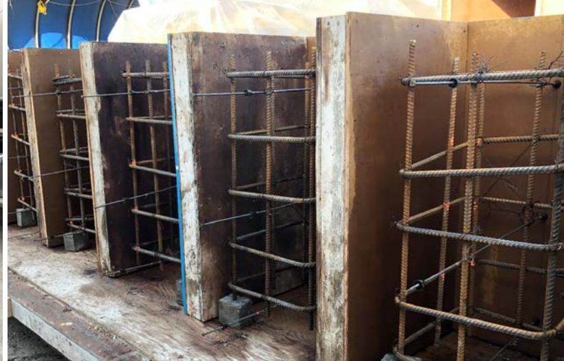
Manufacturing Passenger information Display (PID) foundations for sign posts
