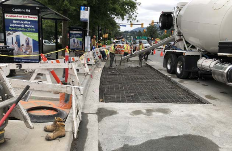
Constructing a new bus pad
