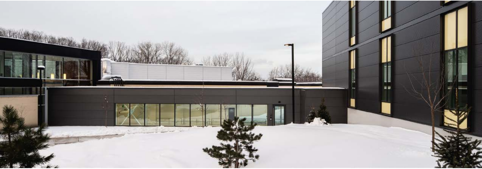
Link from Modular Complex to the Main Hospital
