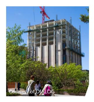
One sustainability-focused challenge was that the existing building featured an inefficient cladding system that led to poor thermal performance. The innovative double-skinned façade greatly improved thermal performance.
