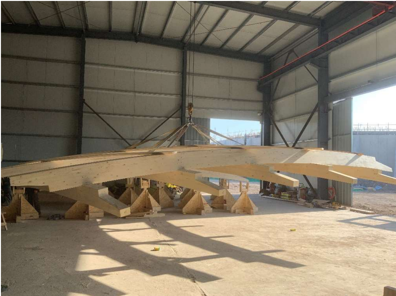
Shop Pre-Assembly of Lattice Panels
