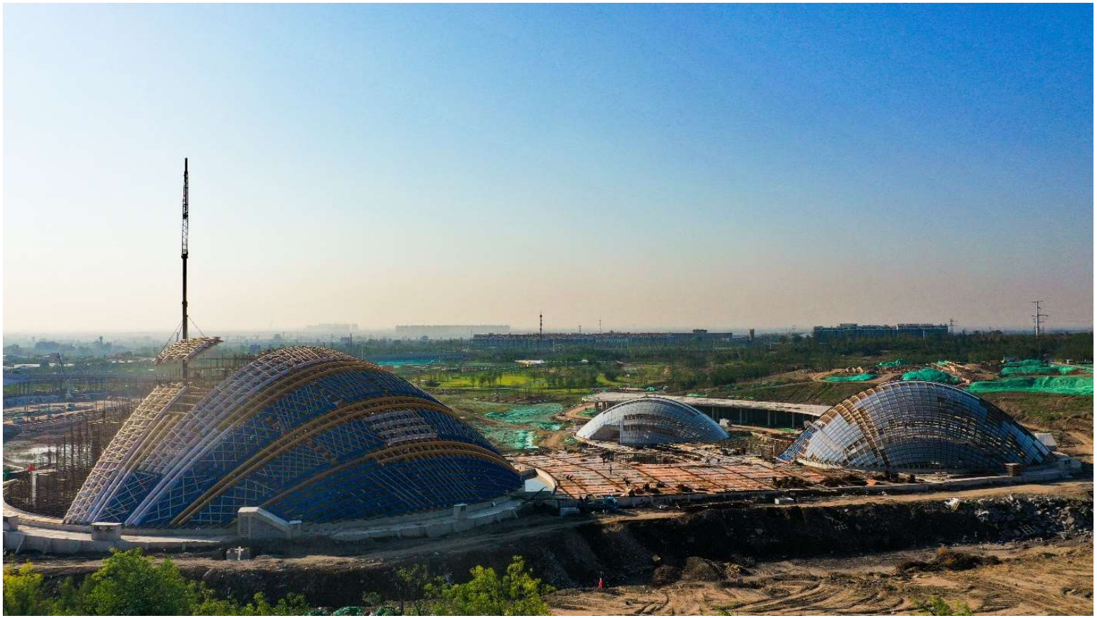
Doubly curved Glulam lattices craned into place. The outside diagonal timbers were temporary, to hold the lattice geometry until erection was complete.
