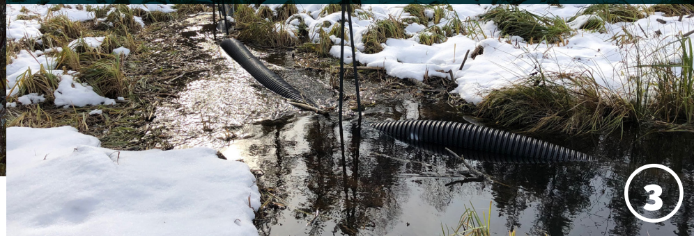
Photo of Beaver Dam #1, with beaver deceivers/water level control devices installed by MTO, November 2019.
