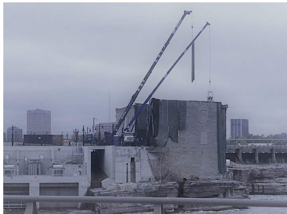
▲ Work in Progress Hoisting the collapsed structure out of the building (JCAL 2018)
