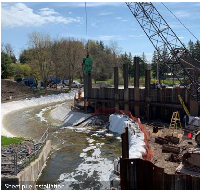
Channel wall reinforcing (Phase 1)
