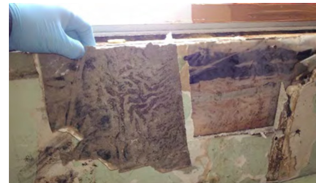
Example of mould formation under damaged windows.
