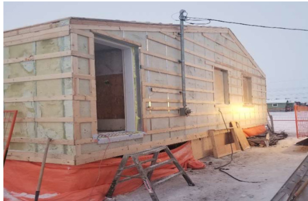
Pilot test unit in Arviat under construction following application of SPF insulation on exterior walls.
