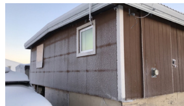
Example of "thermal bridging" through building wood framing.
