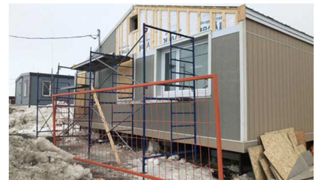
Exterior retrofit near completion - Pilot test unit in Arviat.
