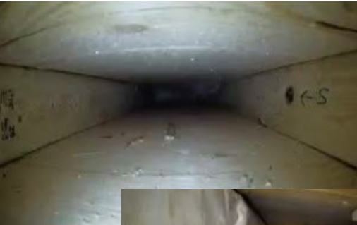
Top: Roof assembly camera image pointed toward soffit vent for snow intrusion monitoring - January, 2020.
