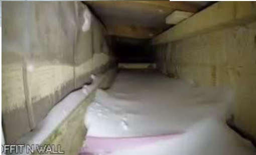
Bottom: Camera mounted within “snow knockout” soffit vent showing snow accumulation. January, 2020.
