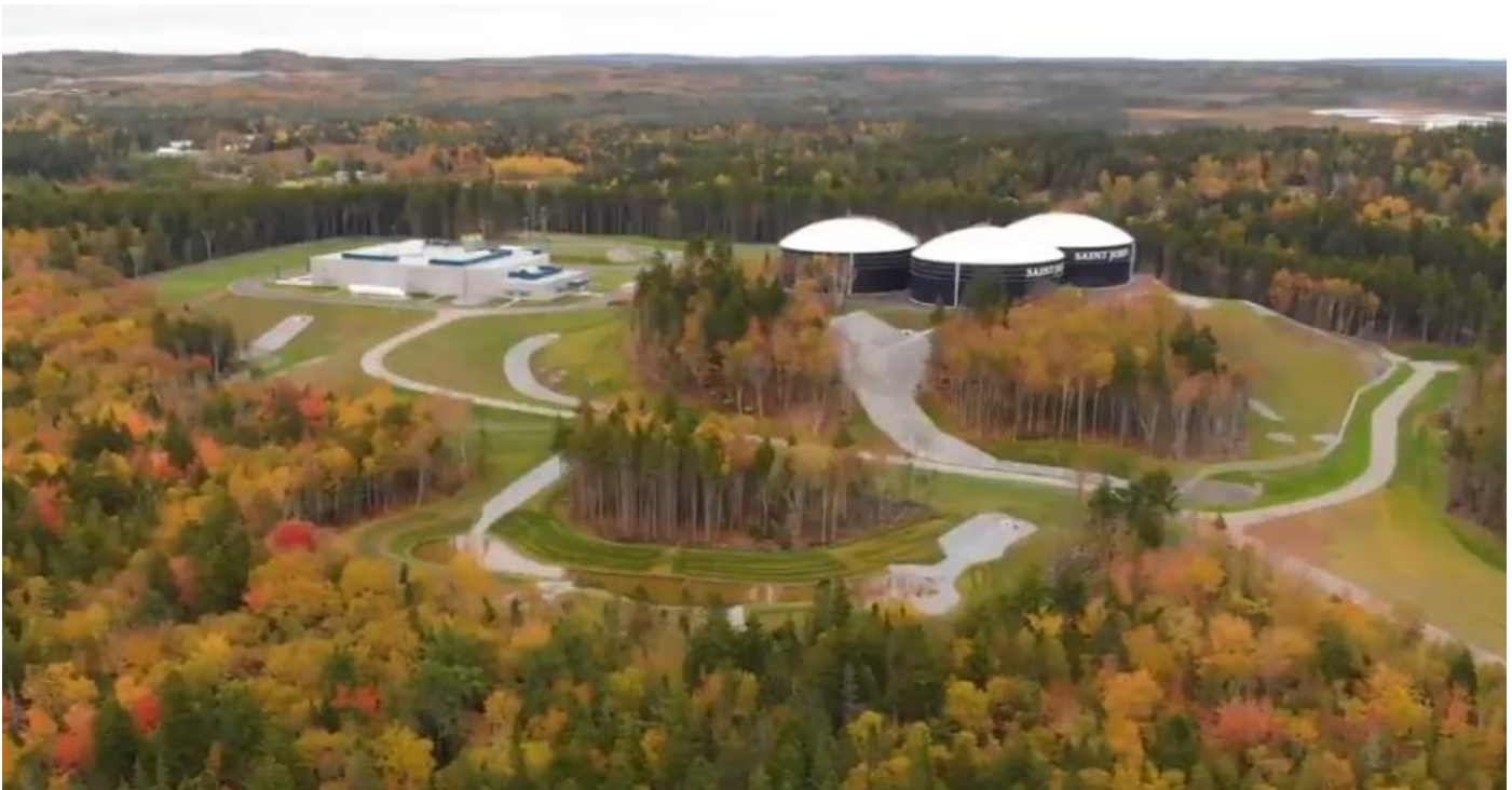
Figure 4: New Water Treatment Plant and Storage Reservoirs
