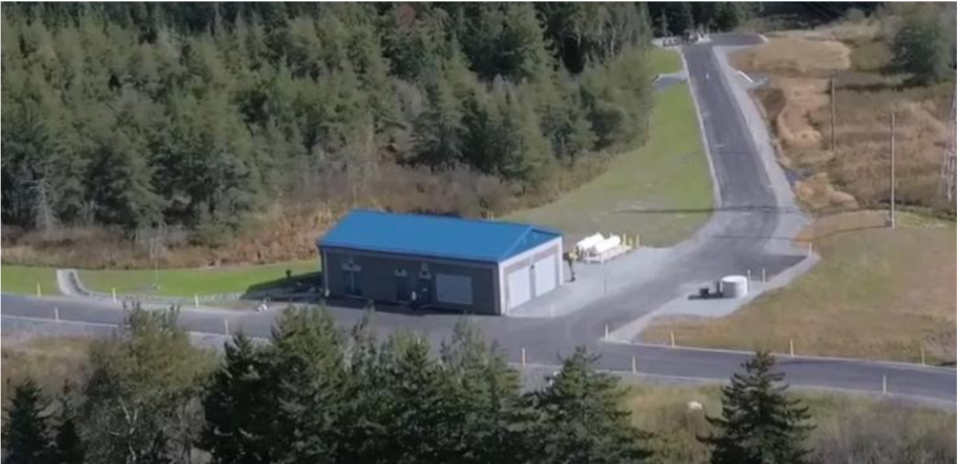
Figure 1: New Groundwater Supply Pumphouse and Standby Electrical Generation located in Island View Heights.
