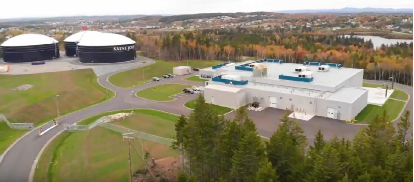
Figure 5: New Water Treatment Plant Storage Reservoirs overlooking Little River Reservoir
