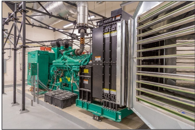
2,000 kW Diesel Generator Set
