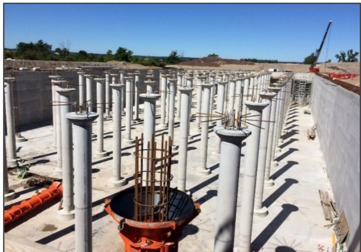
Reservoir Cell Concrete Support Columns
