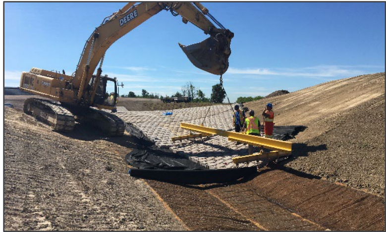
Construction of Overflow Channel
