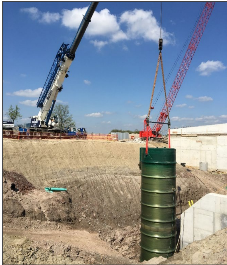
Groundwater Pumping Station Wet Well Placement
