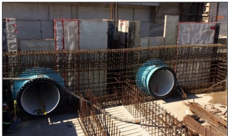
Reservoir Inlet and Flooded Suction Outlet
