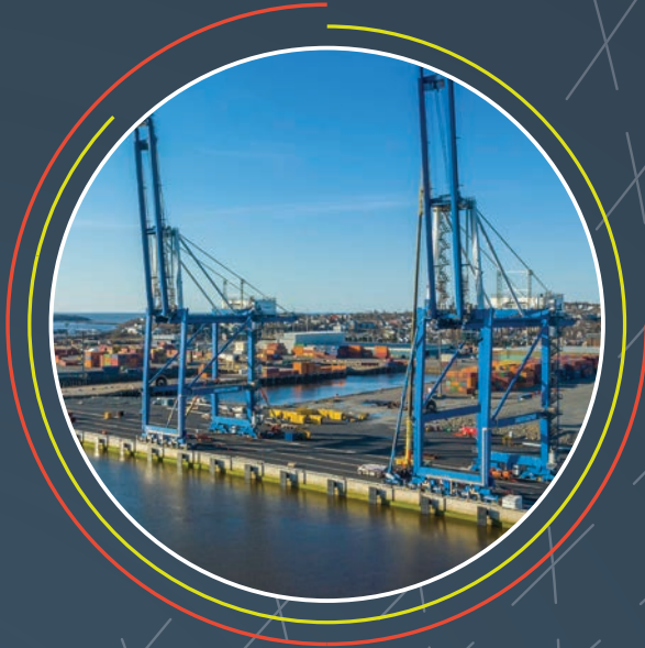
Port Saint John Westside Modernization Project, in New Brunswick
