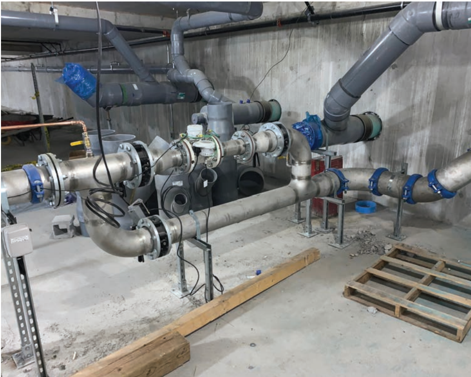
The energy loop required larger-than-normal pipes.
