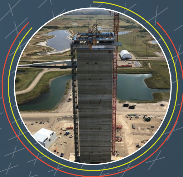
Mosaic K3 Project, South Shaft Headframe, in Saskatchewan
