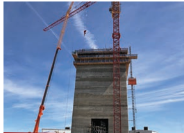
K3 Expansion - South Shaft Headframe
