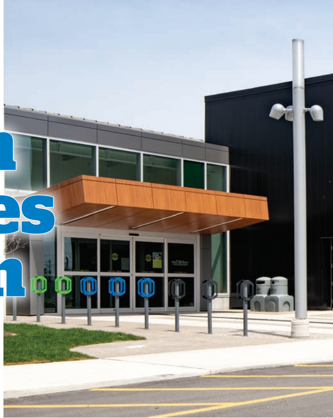
The new Waterloo Public Library features a black solar air heating system.
