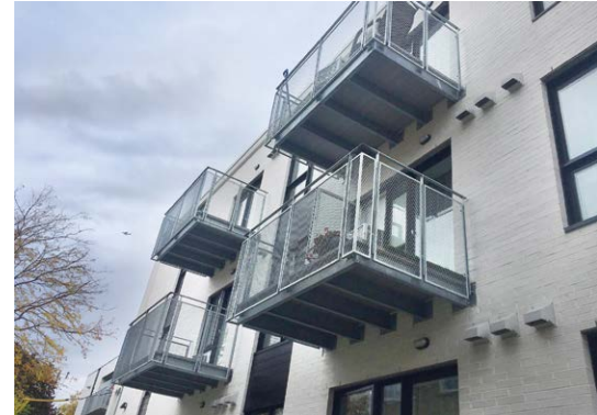
Balconies were retrofitted to the existing structure.
