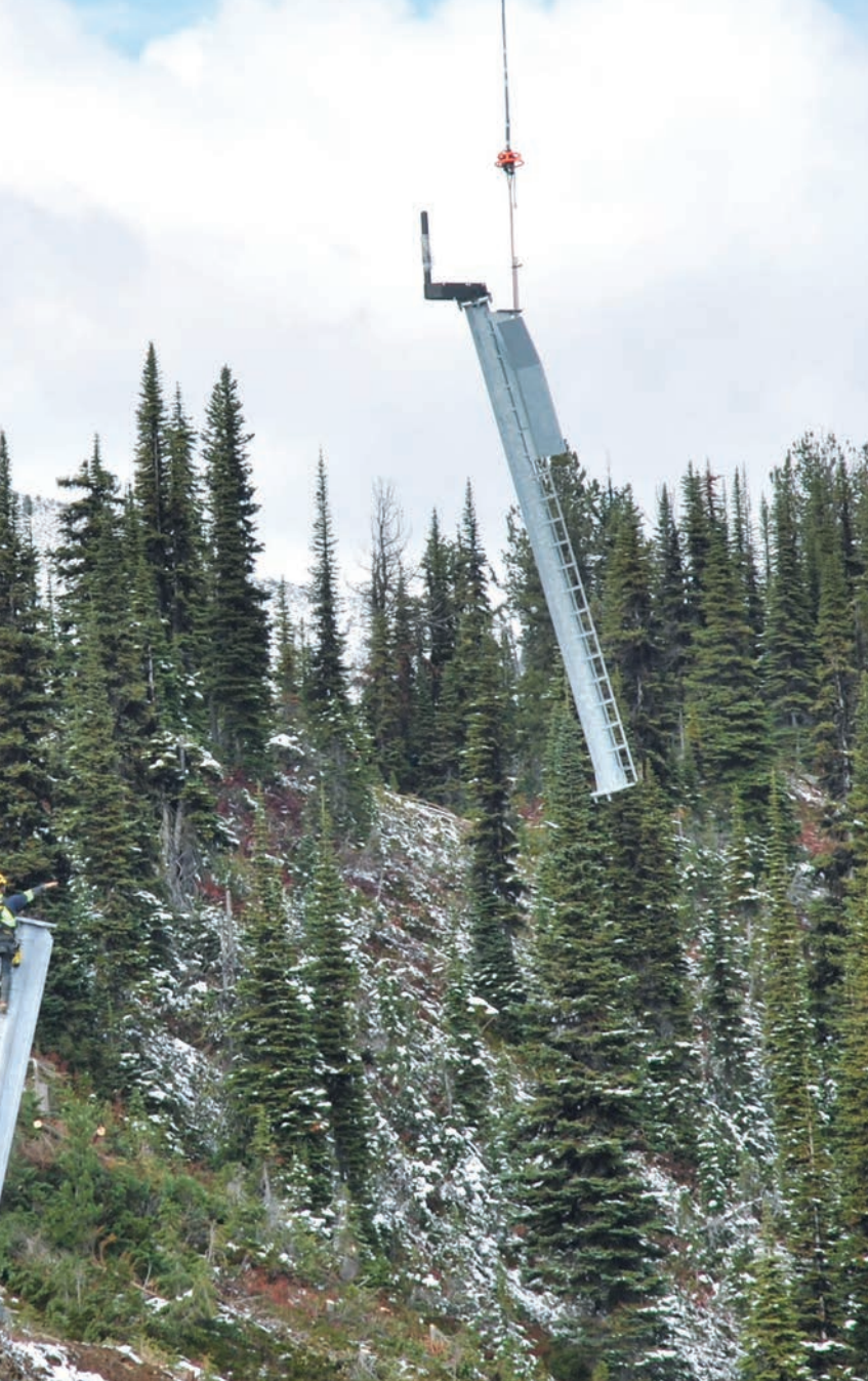
This RACS is solar-powered and its explosives are biodegradable.
