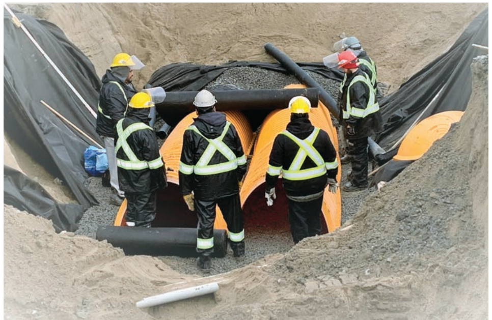
Retention chambers were installed to collect sediments and replenish the groundwater table.
