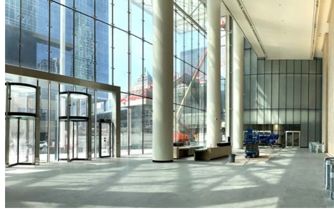
The 24-m tall steel columns in the main lobby support the tower and brace a cable wall.
