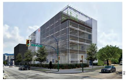
Rendering of the new Fast + Epp headquarters, a four-story mass timber/steel hybrid structure.
