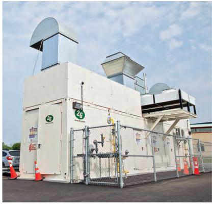
The self-contained 2G combined heat and power plant housing two 265kW natural gas generators.
