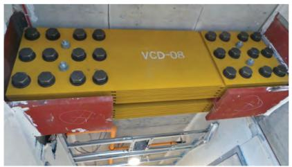
Top: Rigid steel placeholder to be replaced with a VCD unit. Bottom: A VCD unit in place.
