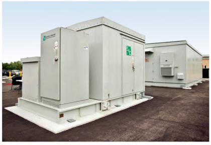
On-site containers house the "brain" of the operation, the S&C GridMaster Microgrid Control System, and the lithium-ion battery energy storage system (BESS).
