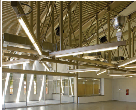
Photograph showing hollow structural steel (HSS) used for the light support framing in lobby area.
