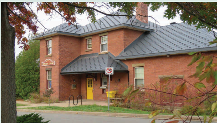
Original diamond shaped asbestos shingles on the old roof.
