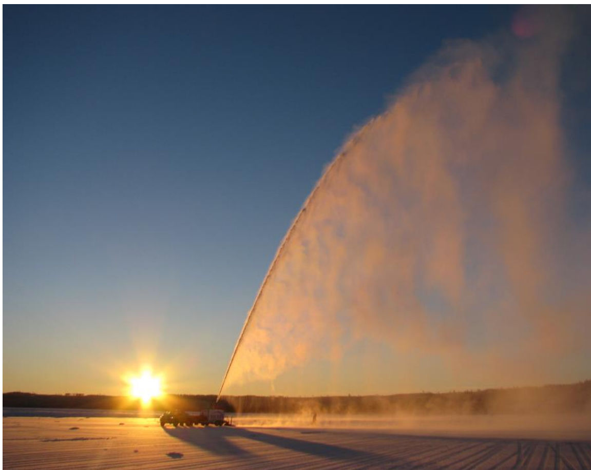
Figure 10: Example of a spray ice operation 7 .
