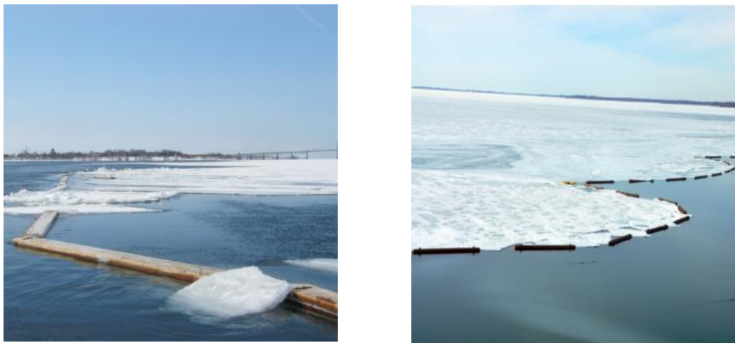
Figure 19: Examples of ice booms used by Ontario Power Generation: Left) timber; right) steel pontoons. 18
