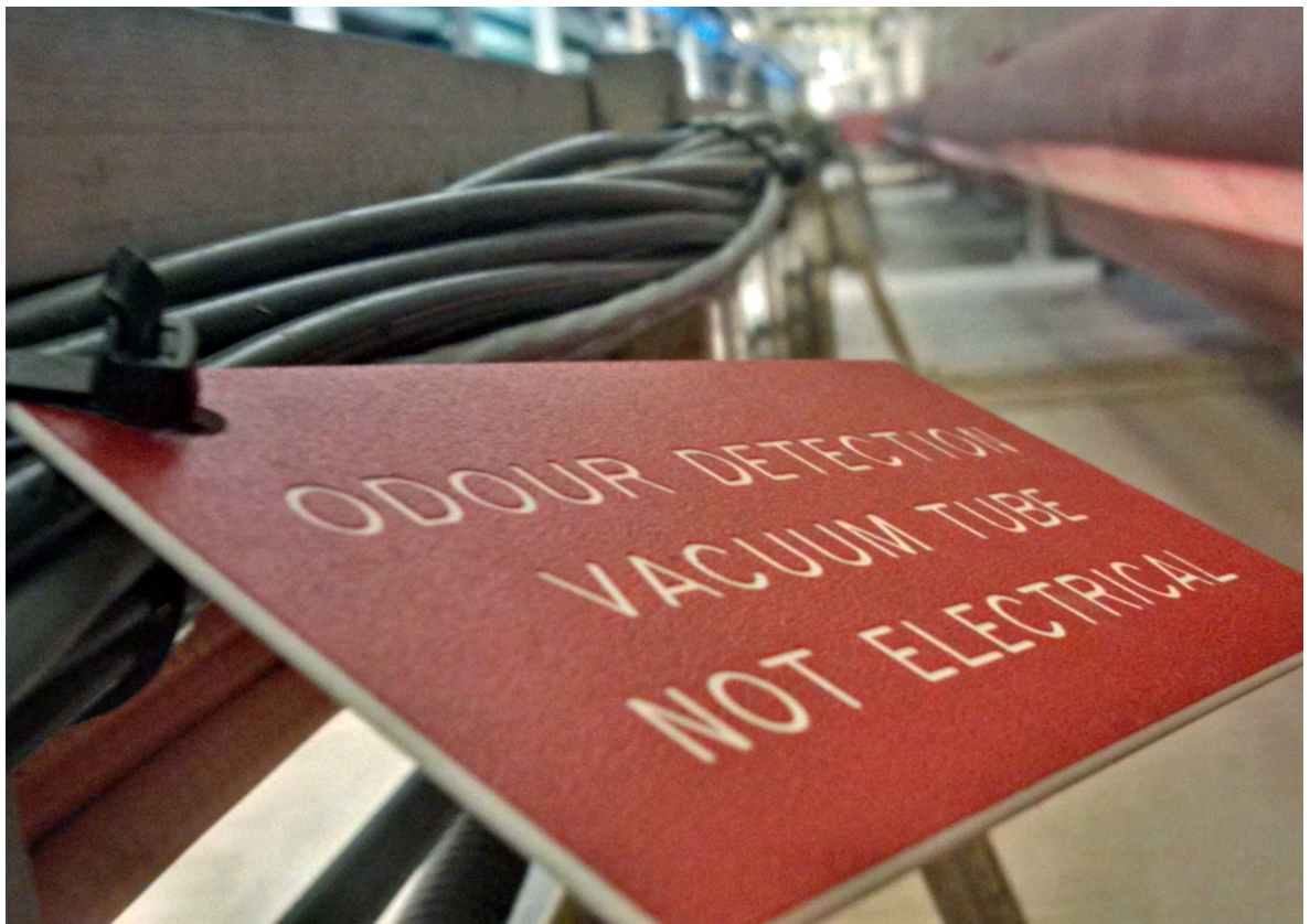
Figure 3 – Airdar Sample Tubing in a FCWWTP Utility Tunnel
