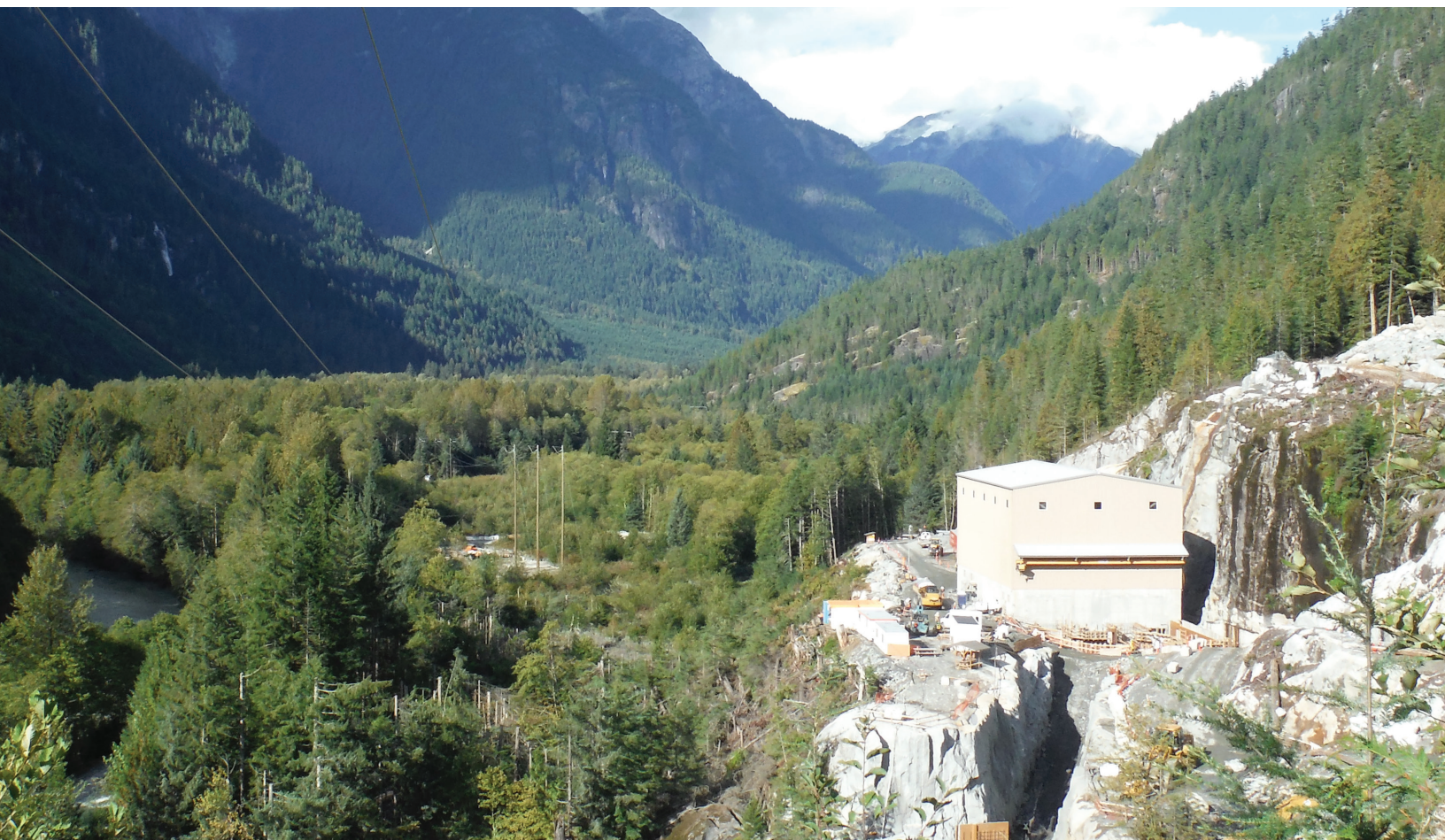
Photo 4: Built on a small elevated rock platform: A surface power station housing two vertical axis pelton turbines
