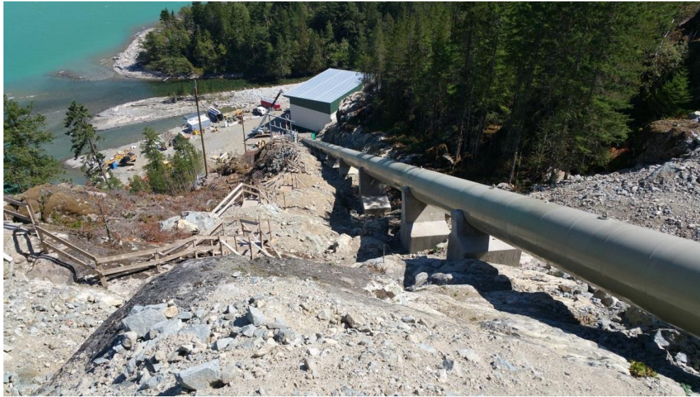
The first 200 m penstock section was installed on a steep slope. It is connected to a powerhouse built on a small ledge excavated into the rock.
