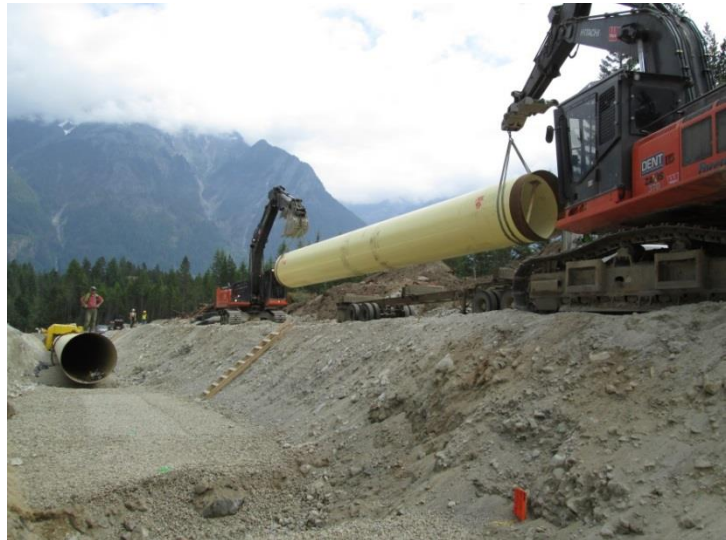
The buried penstock was designed and built to become significantly less visible in just a couple of years.
