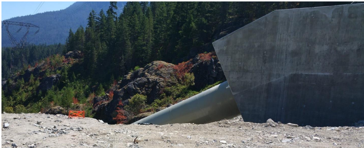
A total of 47 penstock bends, like this one, were required to fit the mountainous topography. On the far left: the power line connecting the facility to the BC Hydro network.
