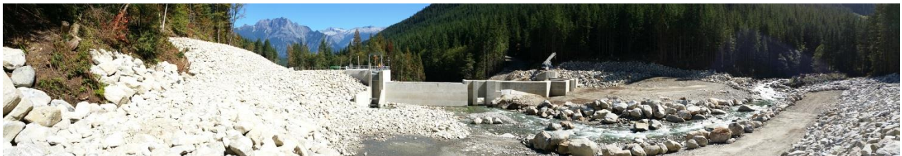
The selected intake (Coanda style) allows fish to migrate downstream without entrainment.
