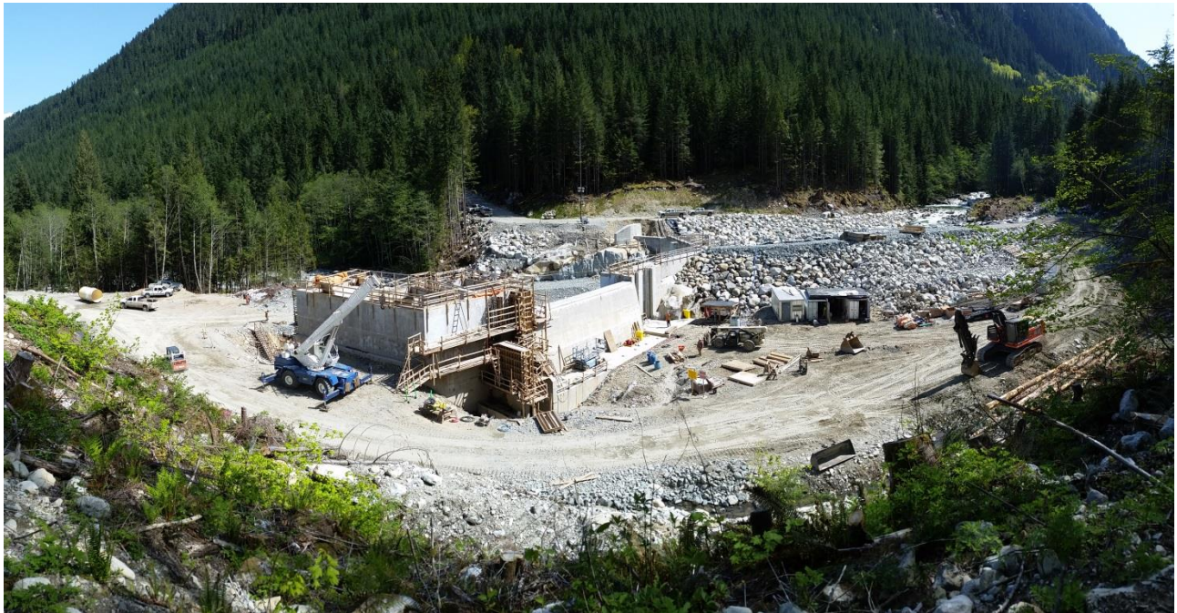
Construction of the intake and weir
