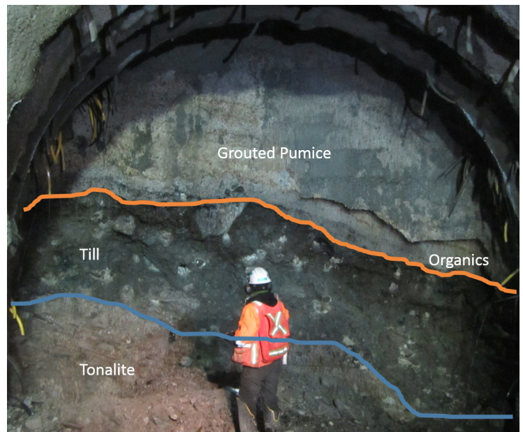
Figure 5 – Mixed face excavation with pumice, organics and till overlying tonalite bedrock.
