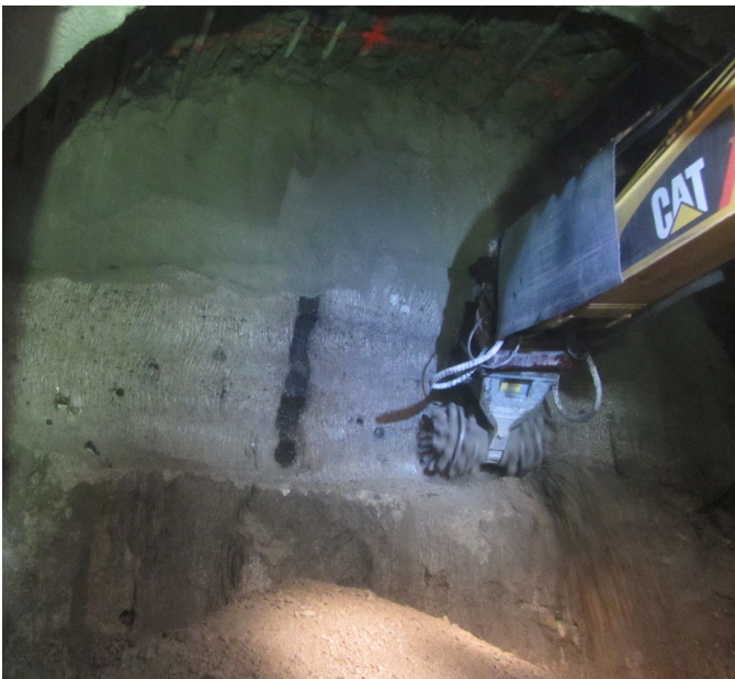
Figure 4 – Grouted pumice deposit containing a burnt tree.
