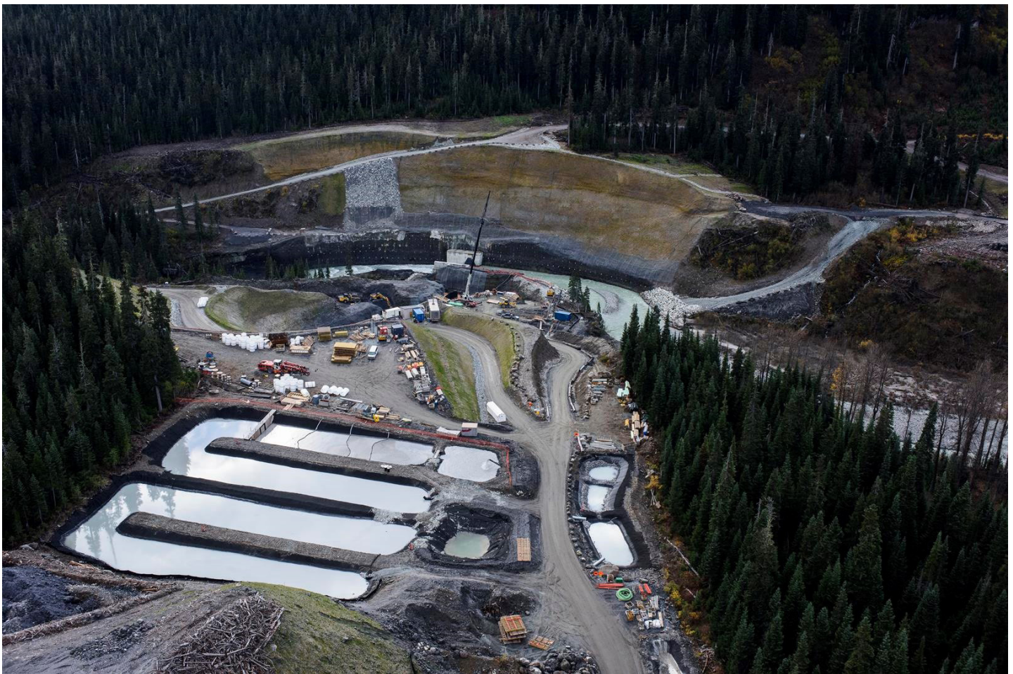
Figure 7 – Upper Lillooet River and construction water management facility at the upstream portal/intake.
