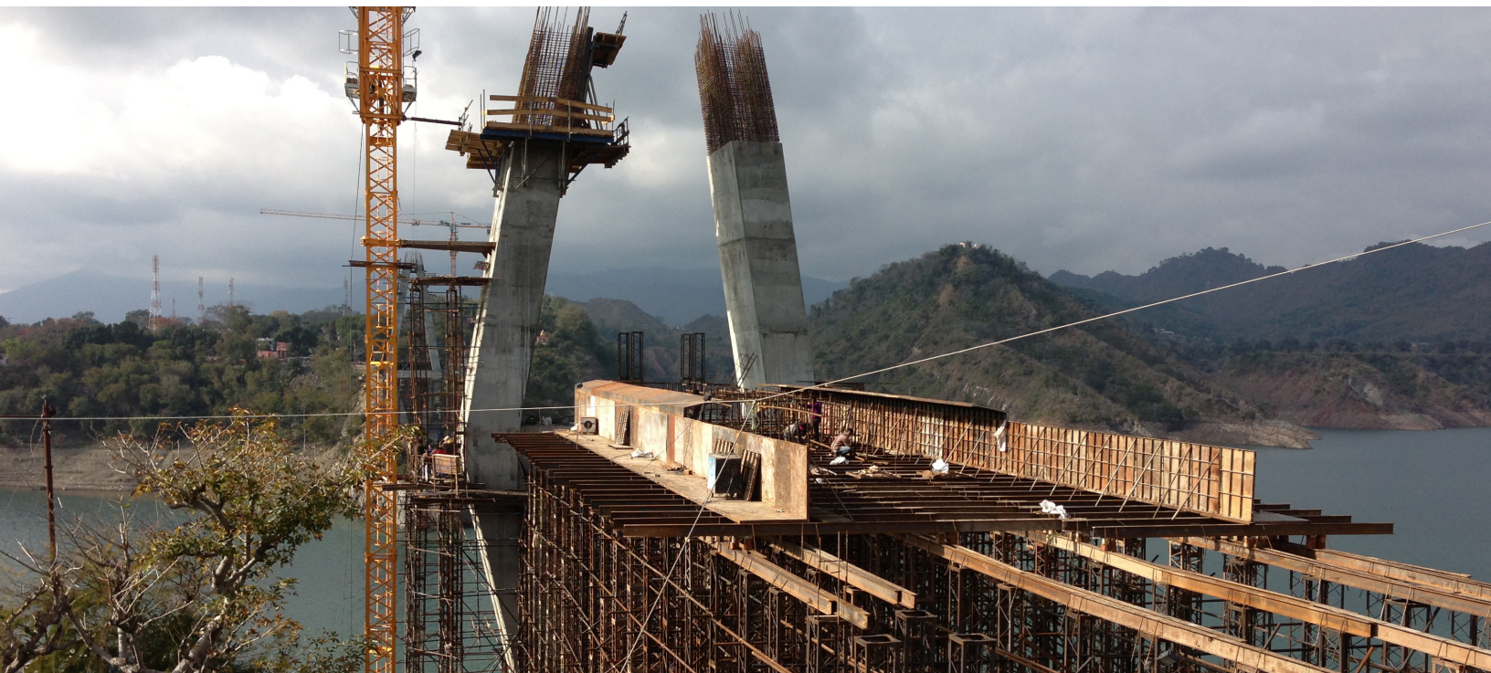
The construction of the side spans and towers.
