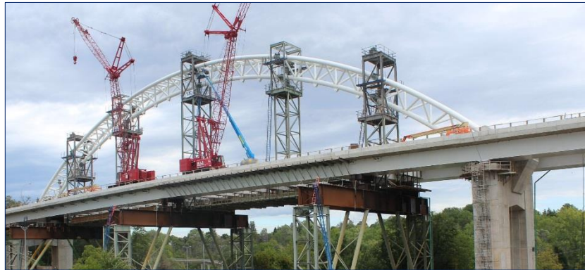
Figure 6 - Arch Shoring Towers Supporting Arch Structure
