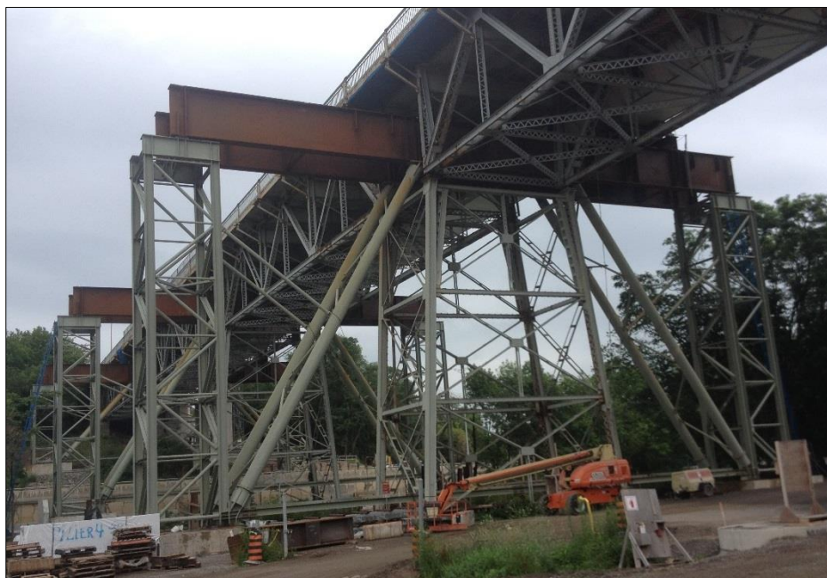
Figure 4 - Temporary Support Towers through Existing Bridge Piers
