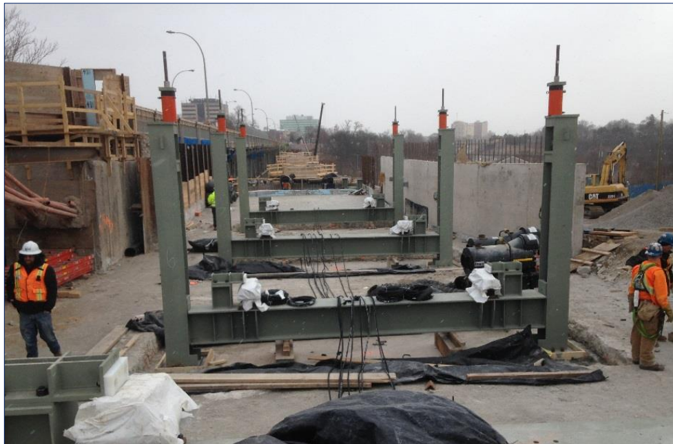
Figure 5 - View from South Approach Through the Box Girder Lifting Frames
