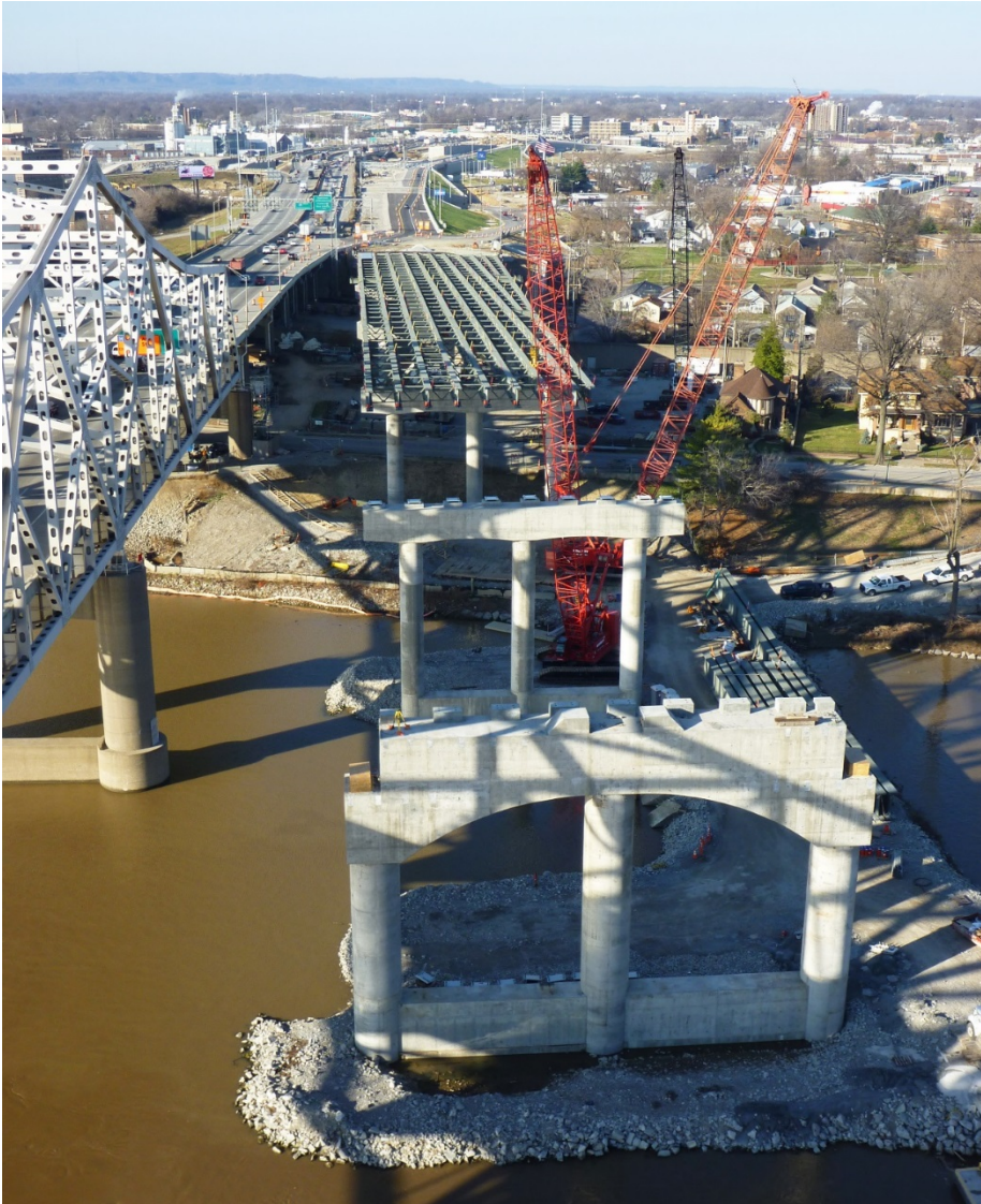
North Anchor Pier and North Approach on Indiana Side.
