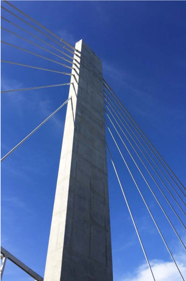
The west leg of Tower 4 with stay cables.
