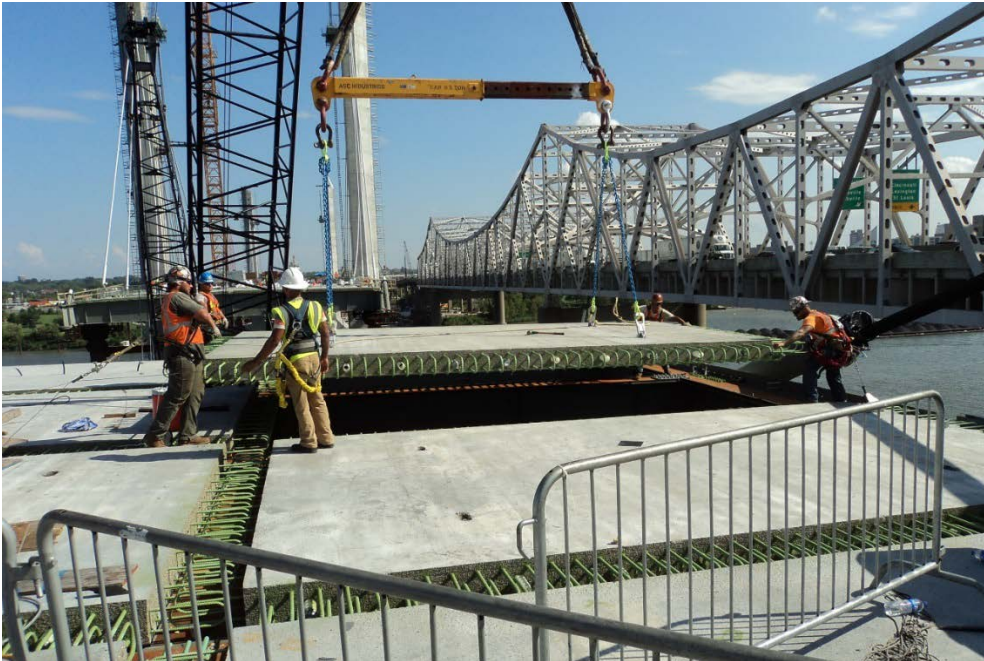
Setting the precast deck panels on the steel superstructure.
