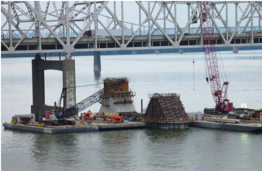
Completed foundation and start of pylon leg.
