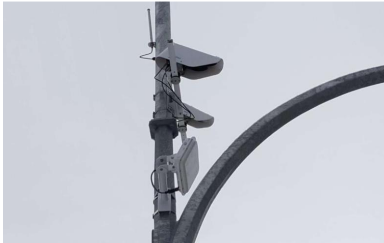
Figure 4: Road Surface Sensors and Traffic Detecting Radar
