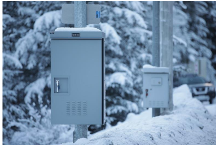
Figure 6: VSLS Cabinets – ruggedized for extreme weather conditions
