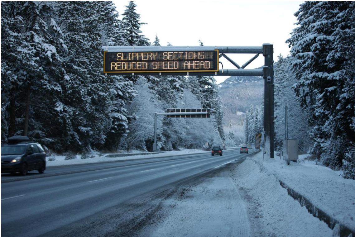
Figure 7: Additional Dynamic Message Signs to warn of changing road conditions and assist drivers to adjust speeds
