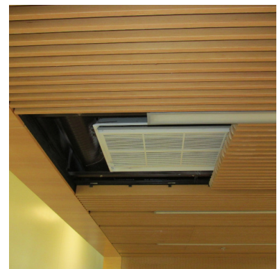
Chilled Beam in Feature Ceiling
