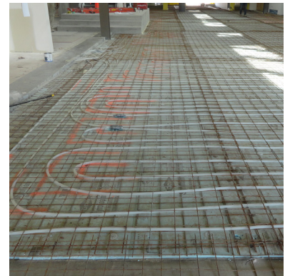
Radiant Heating / Cooling Piping
