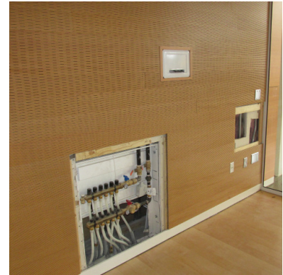
Radiant Piping Manifold
