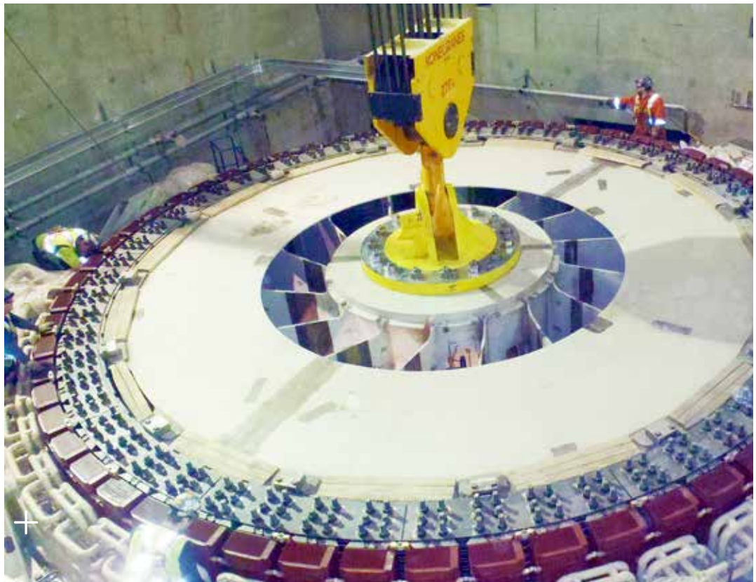
Smoky Falls: Installation of the rotor for Unit 1 in March 2014.
