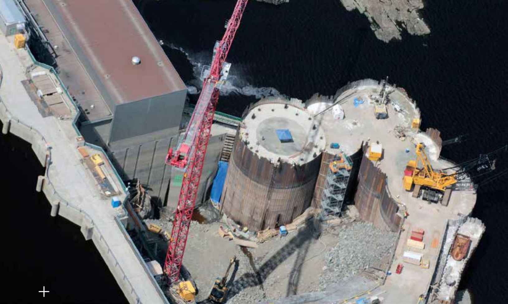
Kipling: Successfully dewatered construction area for Unit 3, adjacent to the operating station.
