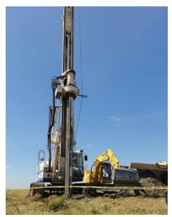
Photo 7 - A typical vertical landfill gas extraction well installation at the Vancouver Landfill. (photo by City of Vancouver).
