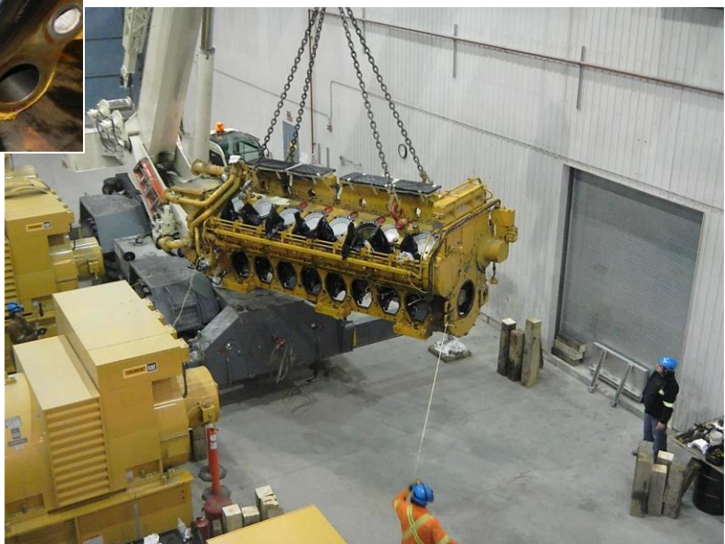
Workers replacing broken engine crankshaft
