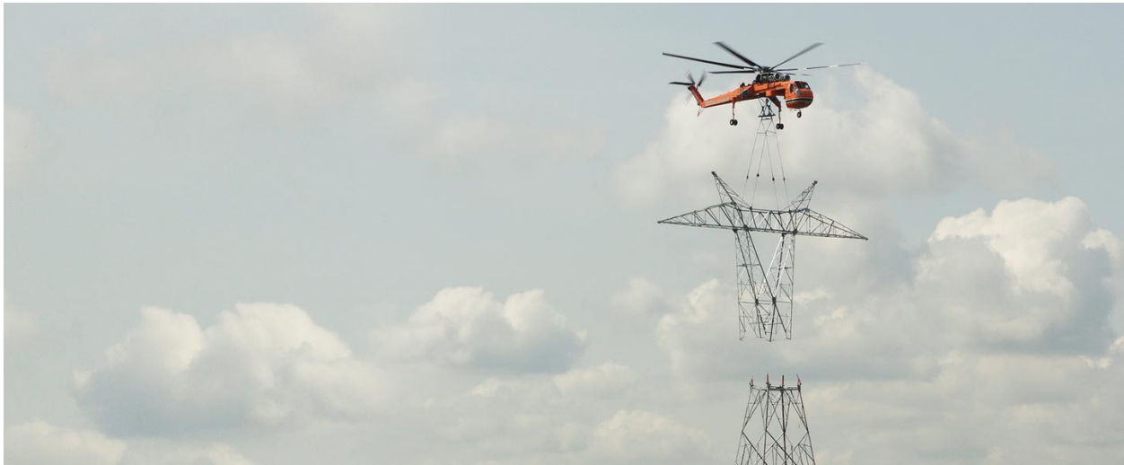
Figure 4: Tower Assembly Using a Helicopter Air Crane
