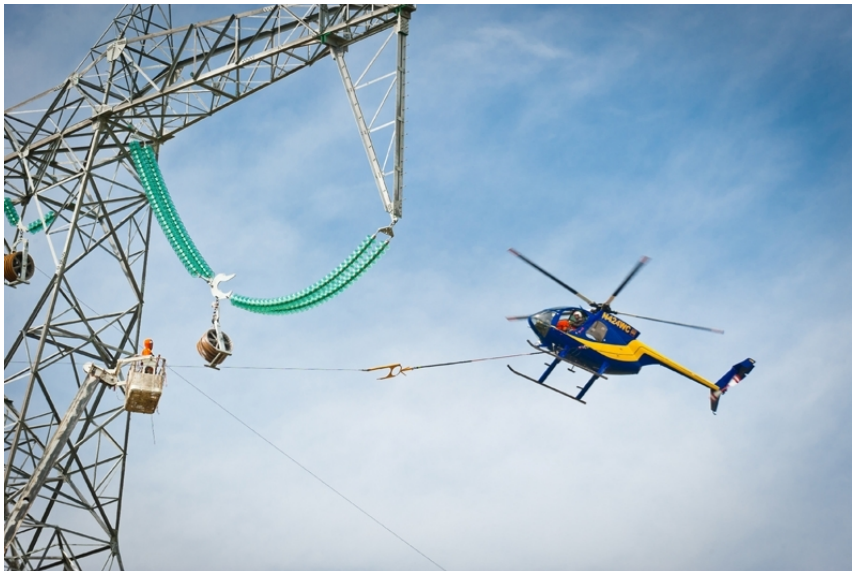
Figure 5: Conductor Stringing using a Helicopter
