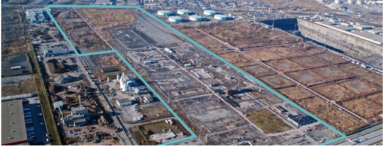
Photo 1: Remediation work zone
