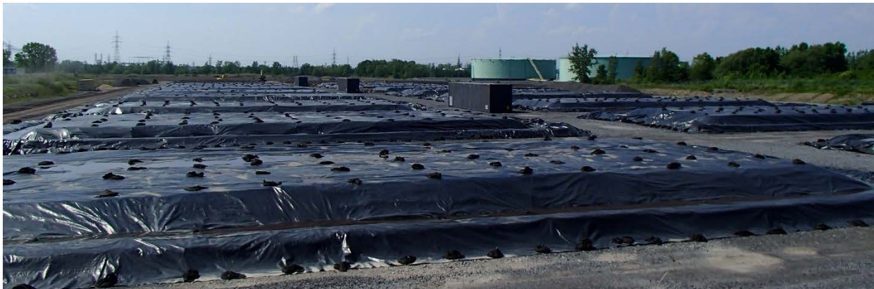
Photo 2: Biopiles designed for the co-composting of contaminated soils.
