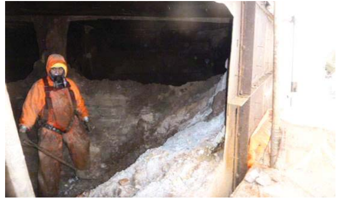
Worker Removing Bulk Arsenic from Inside Flue
