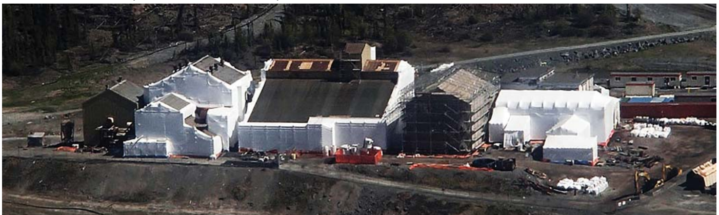
Giant Mine Roaster Aerial View
