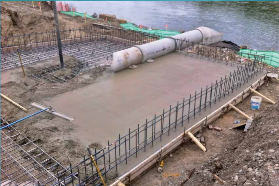
POURING THE BASE SLAB OF THE SUBSURFACE SUPPORT STRUCTURE
