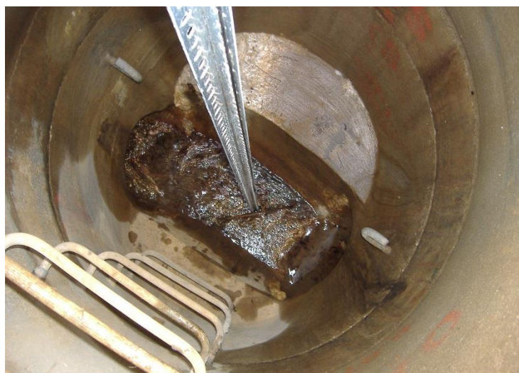
Figure 5 FDC Water Level Monitoring Gauge Installation
