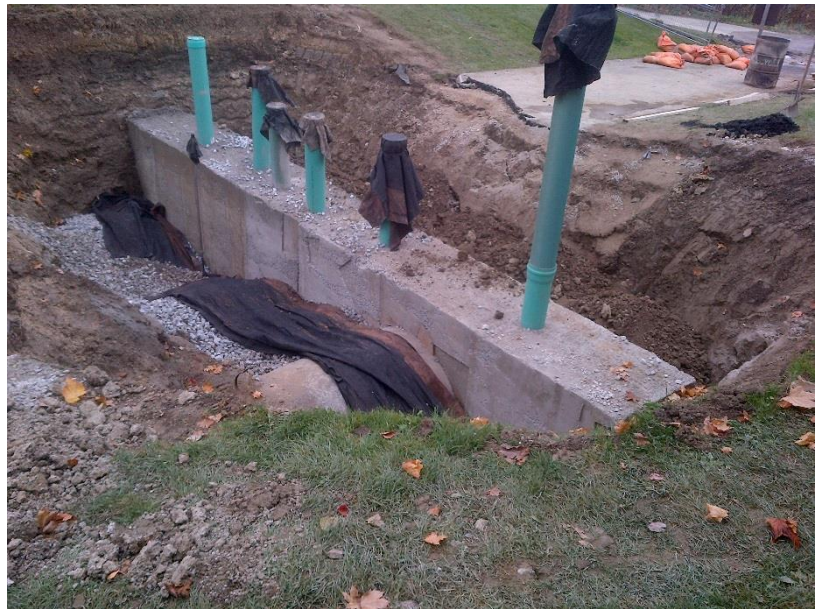
Figure 6 Utility Trench Collar under Construction
