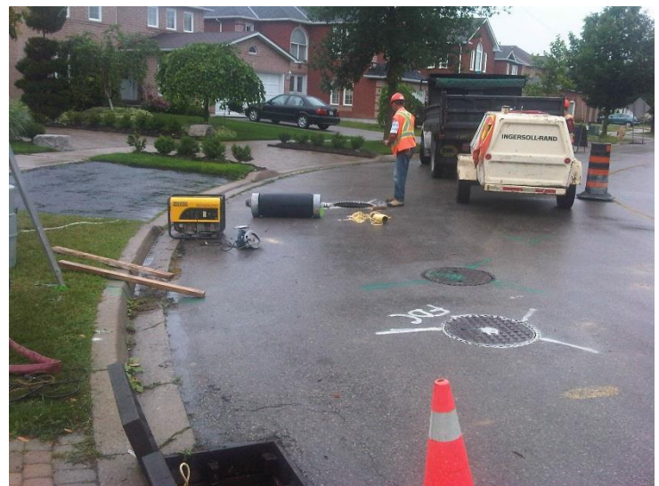
Figure 4 Storm Sewer Leakage Testing Procedure
