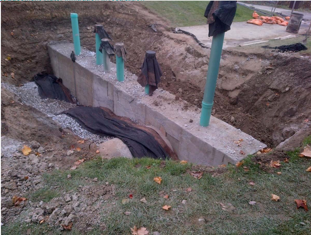
Utility trench collar under construction
