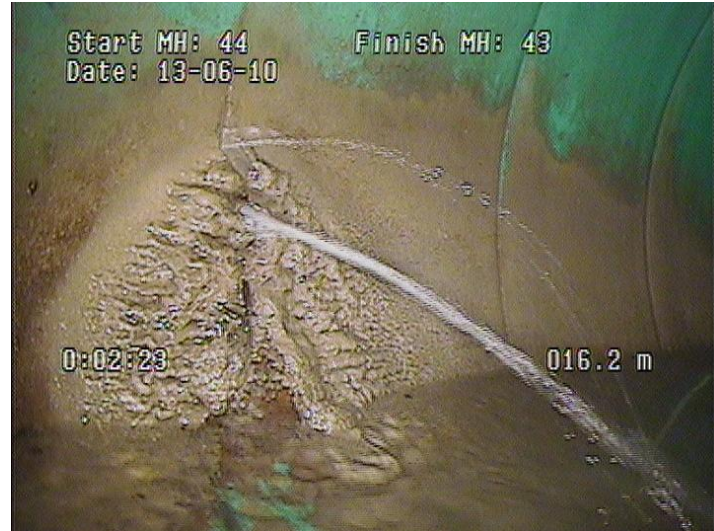
Figure 3 CCTV Inspection of the FDC System Showing Leakage/Infiltration
