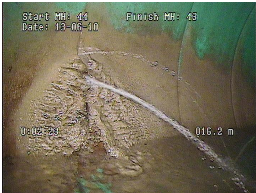
Closed Circuit Television Inspection of the FDC System Showing Leakage/Infiltration
