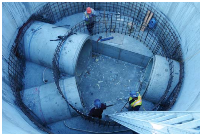
Future Tie-In, connection for expansion
