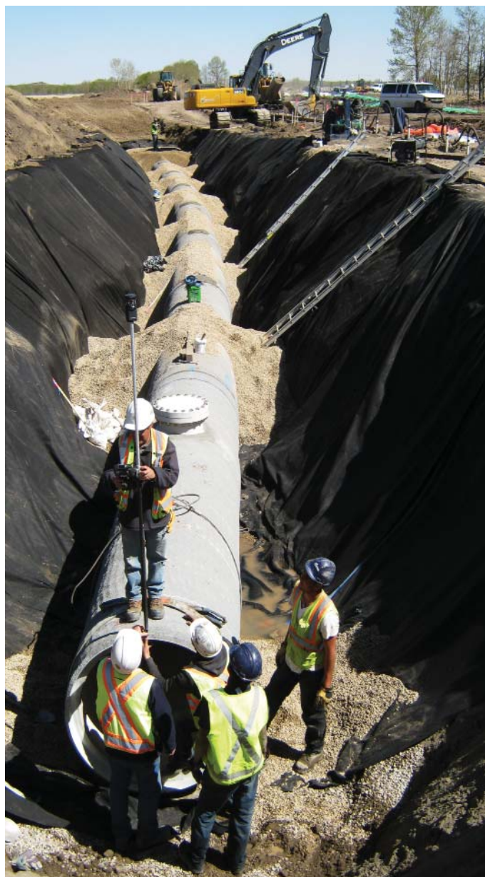
Open trench construction, photo from previous project shows environmental impact
