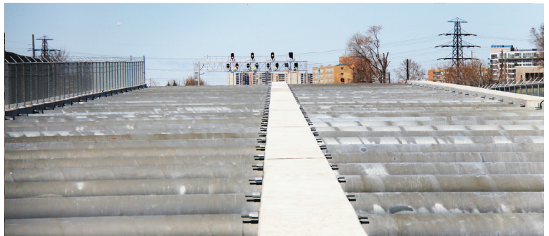
Looking north from the Old Weston Road bridge, the center wall divides the east and west sides of the West Toronto Rail Grade Separation structure.
