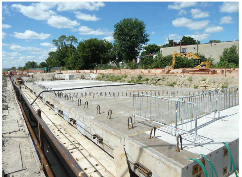
Looking north toward Old Weston Road at the east span of the CP North Toronto Subdivision bridge as it is made ready for sliding south into its final position during a short possession of the CP tracks.
