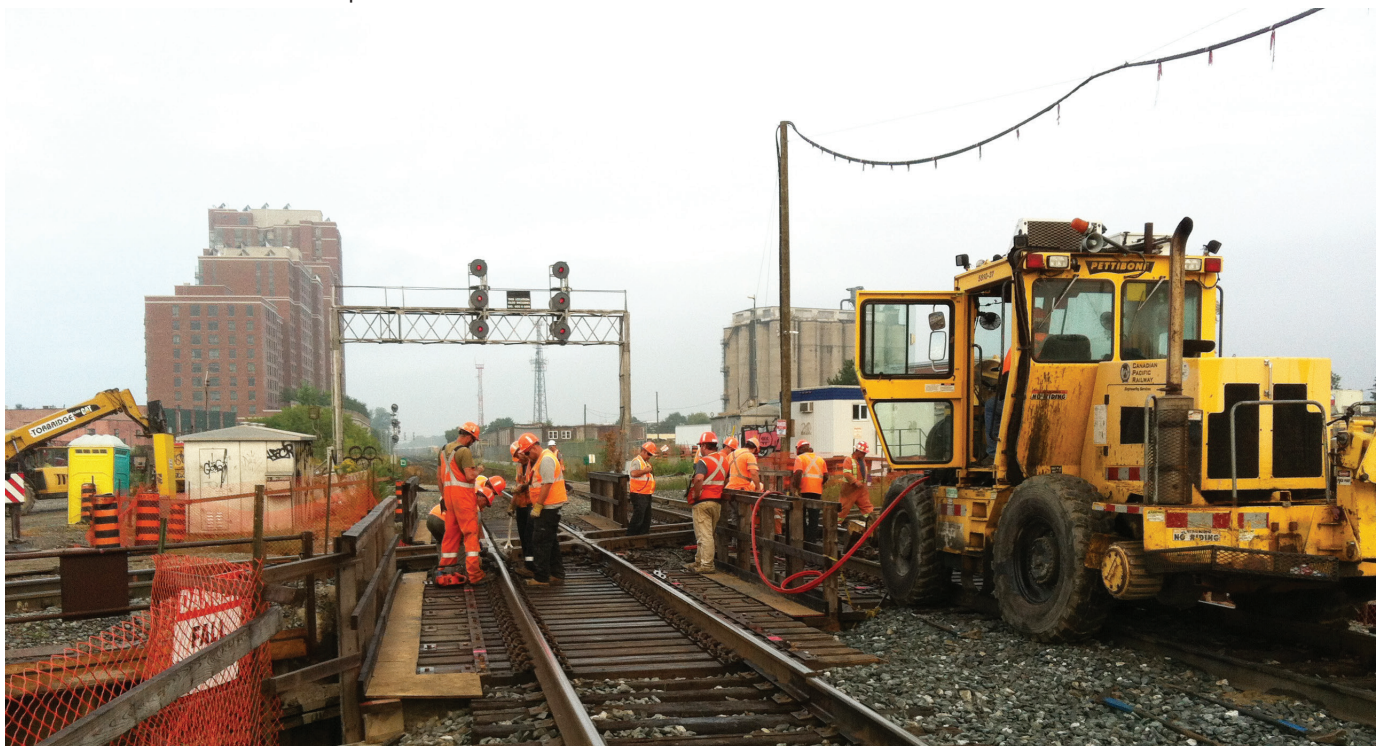
Railway crews maintain track at the temporary, removable bridges carrying the two CP North Toronto Subdivision tracks over the center and west walls of the new depressed corridor. The Metrolinx GO Weston diversion track and its “diamond” crossings are visible in the background.
