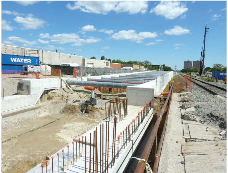
Looking south from the CP North Toronto Subdivision bridge location showing east corridor construction well advanced, including the stepped wall caps in the foreground being made ready to receive the east bridge span when it is slid into position.
