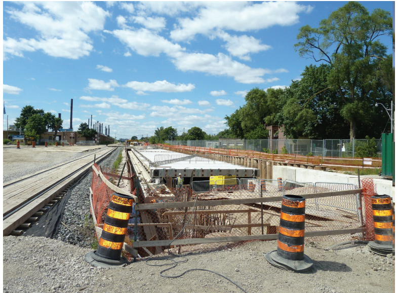
Looking north toward Old Weston Road, the east span of the Old Weston Road bridge is made ready for sliding north into its final position during a short possession of the CP connection track.
