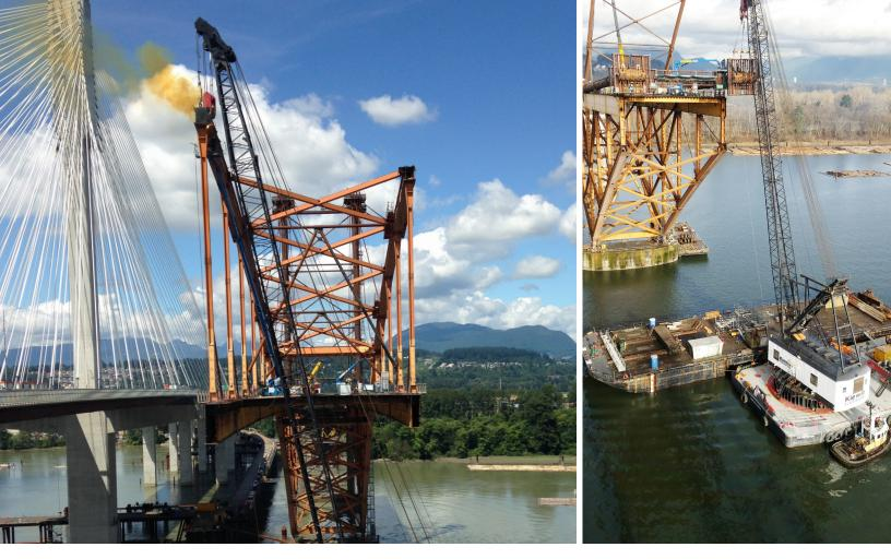
Pieces of the bridge were carefully removed by crane and lowered onto a barge for recycling. Note the proximity to the new bridge.
