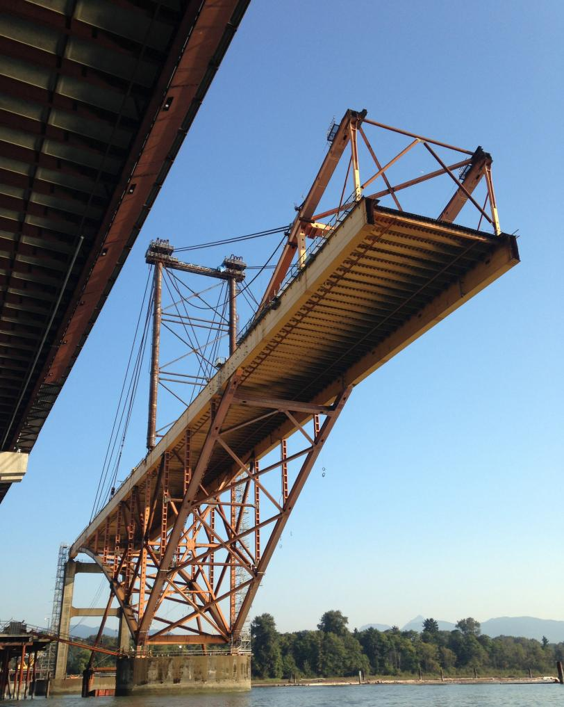
Temporary cable-stayed cantilever system.
