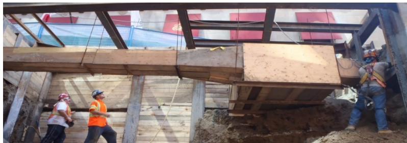
Supporting Utilities During Construction
