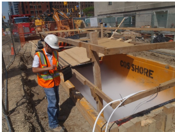
Freezing of Hydro One Transmission Circuit with Nitro Glycerin
